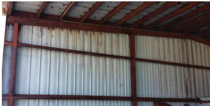
**Figure 4.2.** Rusted hangar not usable for aircraft storage. Source: Delta Airport Consultants, Inc.
