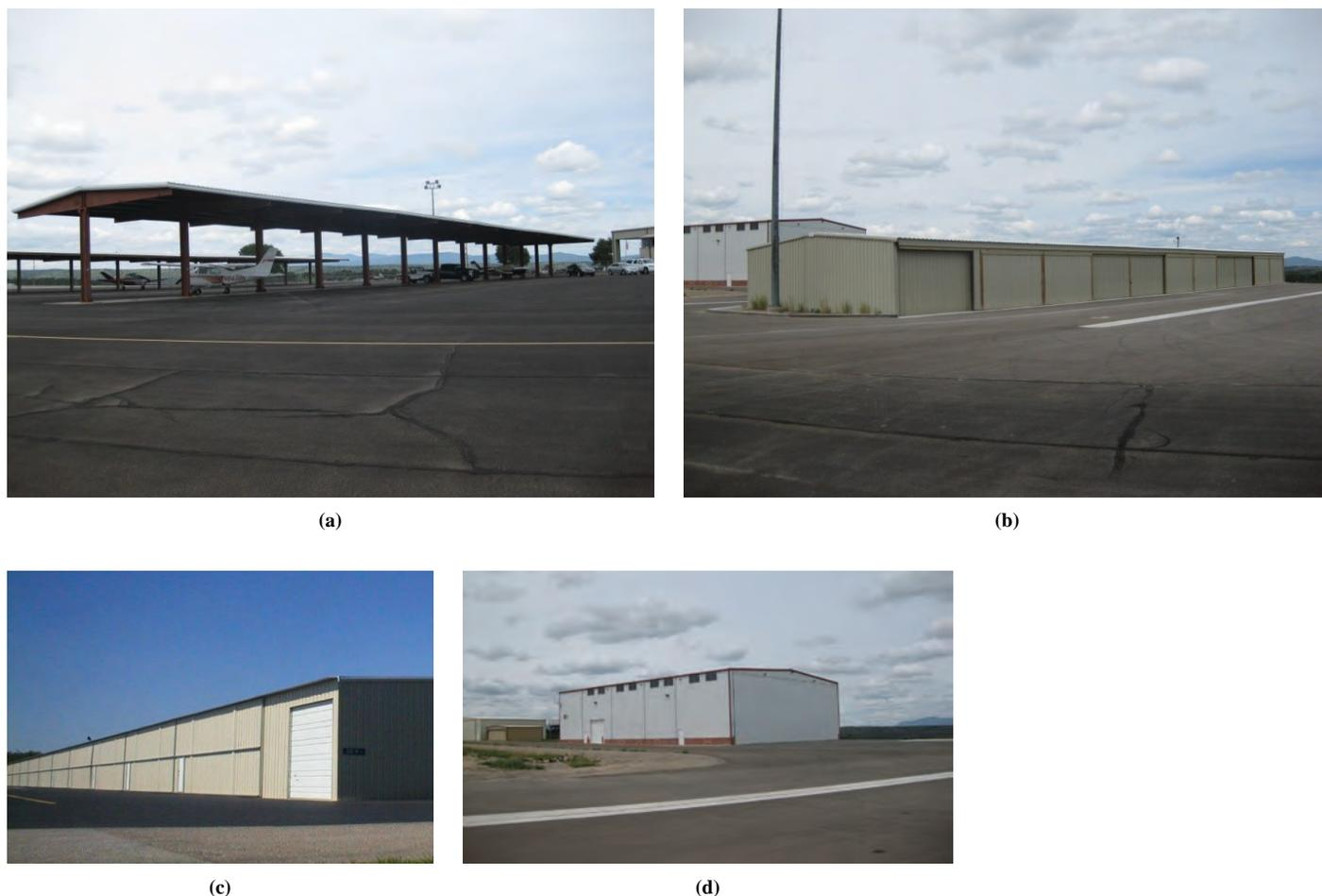
**Figure 3.8. Hangar types: (a) shade, (b) T with simple door, (c) T with bi-fold door, and (d) box. Source: Delta Airport Consultants, Inc.**
