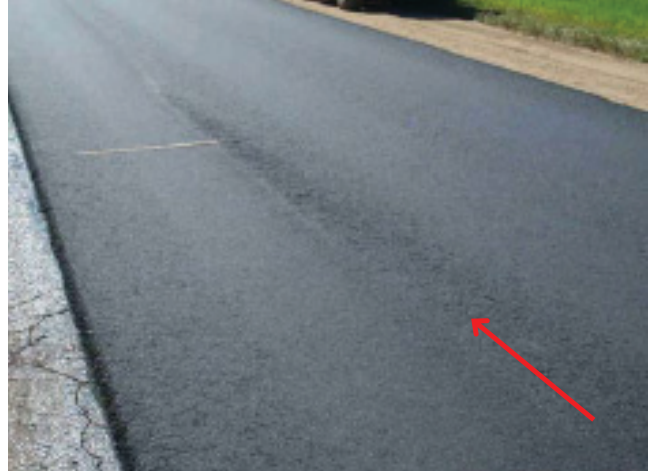
FIGURE 6 Example of longitudinal segregation on one side [Source: Adams et al. (2001)].
