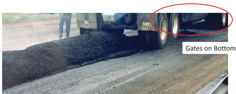
Belly dumps drop mix when the gates at the bottom of the truck bed deposit mix into a windrow on the exiting surface
