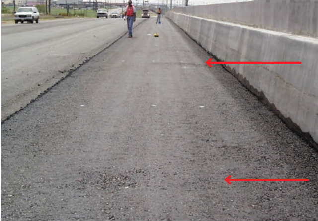
FIGURE 3 Example of end-of-truck segregation [Source: Stroup-Gardiner and Brown (2000)].
