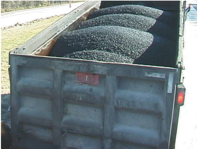
FIGURE 46 Loading large haul trucks with multiple drops [Source: Warren (2012)].
