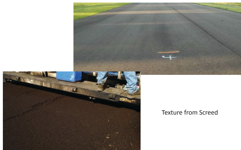
FIGURE 63 Example of large aggregates leaving tears in mat from being dragged by screed [Source: (top) Warren (2012); (bottom) Stroup-Gardiner (2014)].
