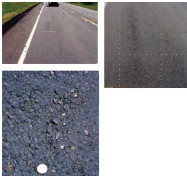
FIGURE 9 Example of slight level of segregation [Source: Gavin and Heath (2002)].
