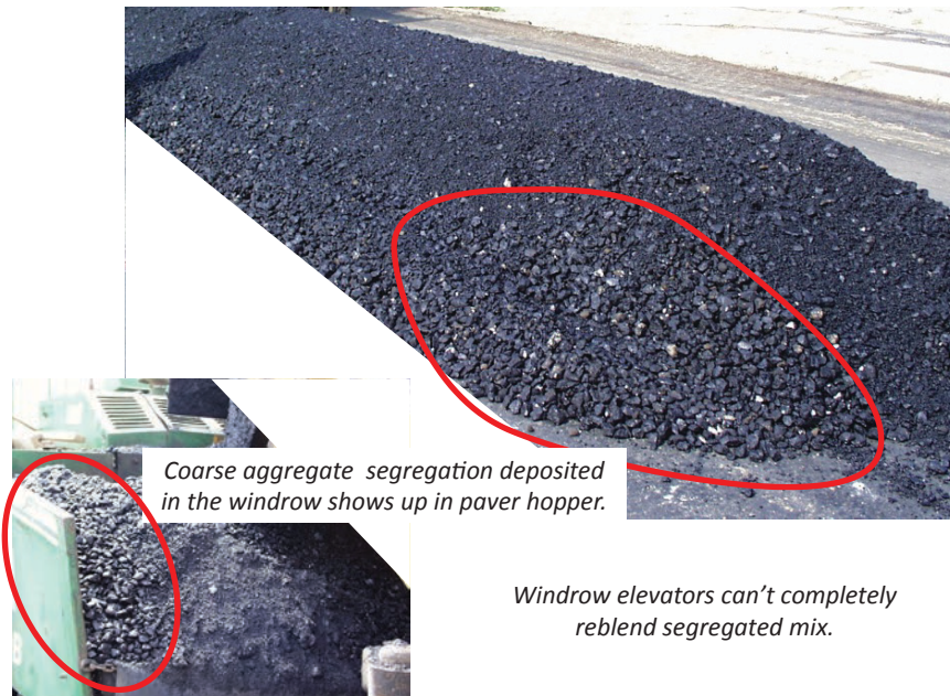
FIGURE 52 Segregated mix in the windrow can still remain segregated when it gets to the paver hopper [Source: Stroup-Gardiner (2014)].
