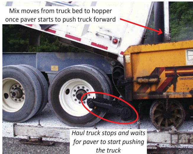
FIGURE 47 Transferring asphalt mix to the paver hopper [Source: Stroup-Gardiner (2014)].
