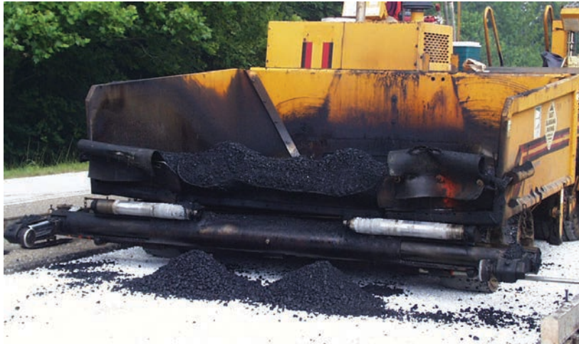
If left, spills create a bump in lane and leave mix to get cold. Cold mix can result in low densities.
