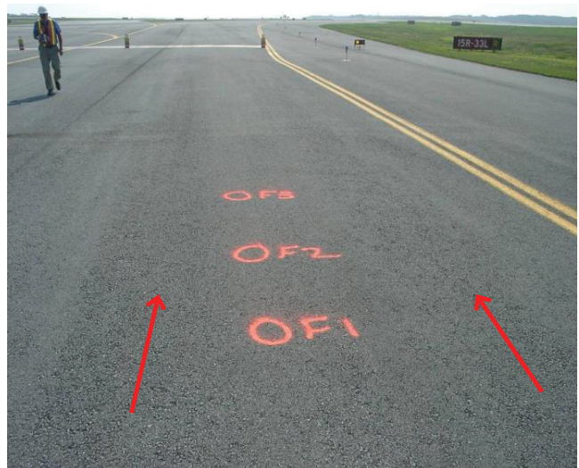
FIGURE 7 Example of longitudinal segregation, both sides [Source: Murphy (2012a)].
