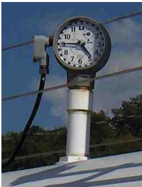
FIGURE 7 Fuel tank float type clock measurement gauge. (Courtesy: S. Quilty, SMQ Airport Services.)
