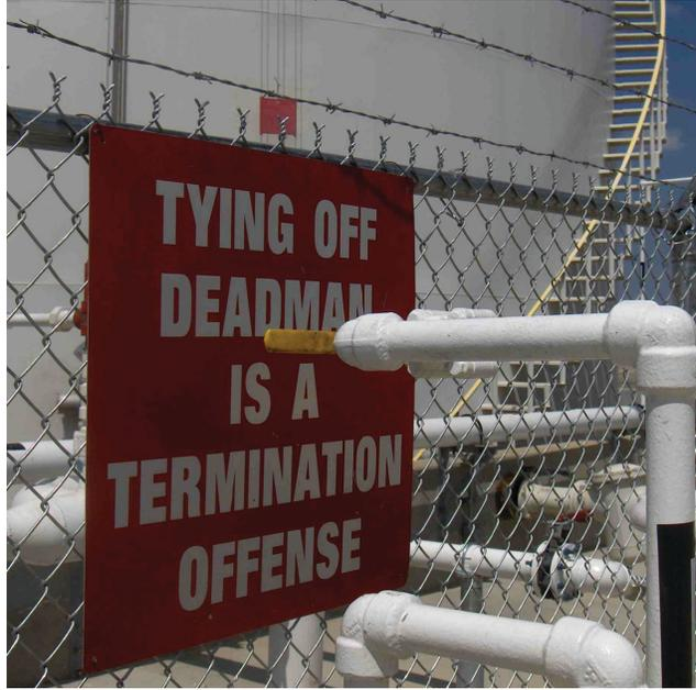
FIGURE 27 Sign designed to deter an unsafe fuel loading practice. (Courtesy: S. Quilty, SMQ Airport Services.)
