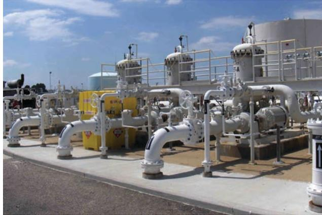
FIGURE 12 Example of parallel pumps for hydrant fuel system. (Courtesy: S. Quilty, SMQ Airport Services.)
