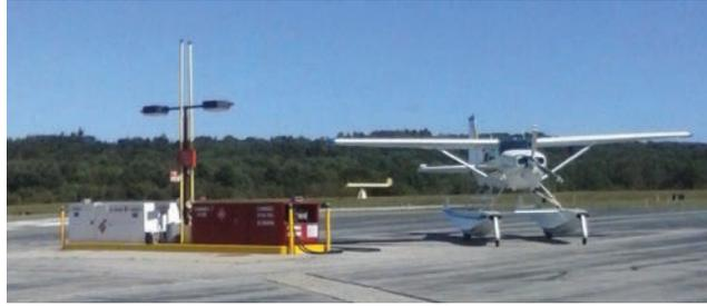
FIGURE 14 Typical fuel island arrangement with low-profile cabinets. (Courtesy: R. Lanman, Auburn–Lewiston Airport, Maine.)
