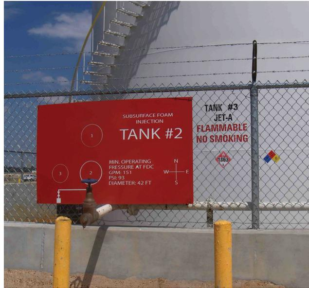
FIGURE 6 Foam suppression inlet point for aboveground tanks. (Courtesy: S. Quilty, SMQ Airport Services.)
