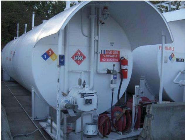
FIGURE 5 Example of a modular fuel tank. (Courtesy: S. Quilty, SMQ Airport Services.)
