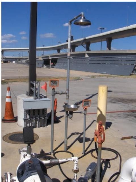
FIGURE 24 Example of eye wash and water deluge system at a fuel loading area. (Courtesy: SMQ Airport Services.)
