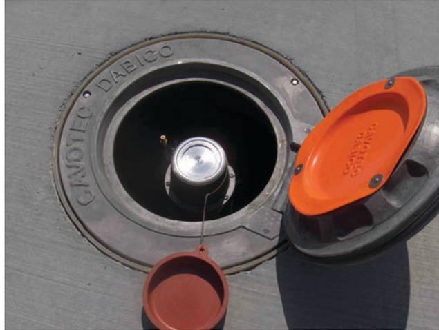
FIGURE 9 Example of a hydrant pit connection on a terminal ramp. (Courtesy: S. Quilty, SMQ Airport Services.)
