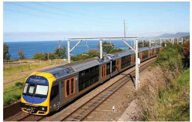
Electric multiple-unit (EMU) train (Australian OSCAR)
