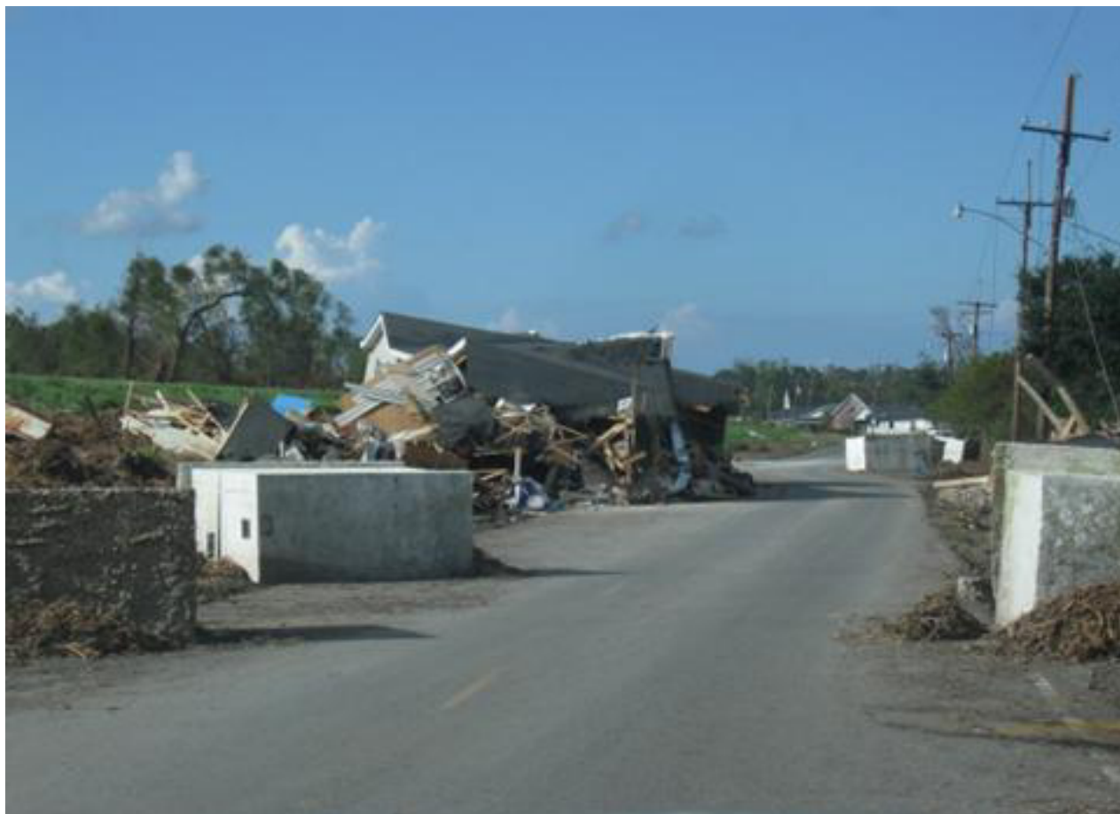
FIGURE D - 65: Hurricane Isaac, 2012 – Debris on LA 39, Braithwaite. Courtesy: Louisiana DOTD.
