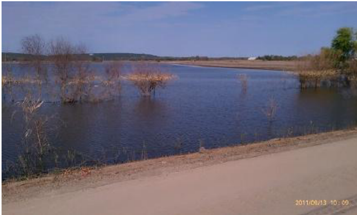
FIGURE D - 7: General Condition of Ditches. Courtesy: Iowa DOT.
