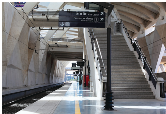
Figure 12-3. The air/rail station platforms at Lyon are largely empty. Source: www.Shutterstock.com . Copyright: procasson Frederic.
