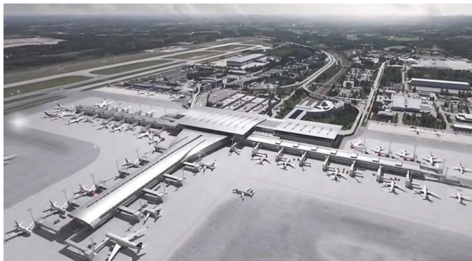
Figure 12-5. At Oslo Airport, the rail alignment under the terminal (center) and under the airside area allows through-routed intercity service. Source: Oslo Airport.
