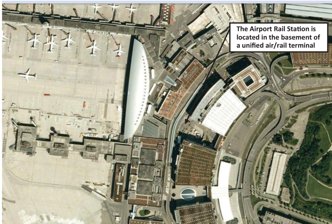
Figure 2-16. At the Zurich airport, the rail station is located within the unified air/rail complex. Imagery © DigitalGlobe, GeoContent, Map data © 2011 Google.
