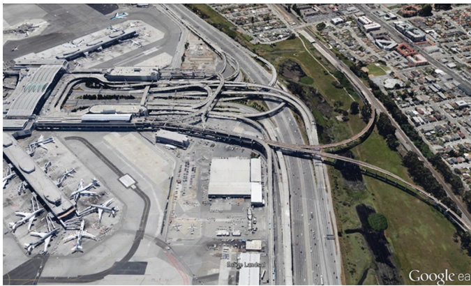
Figure 7.3. Location of BART tracks in and out of SFO. Imagery © Landsat, Google Earth.
