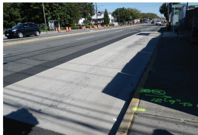
FIGURE 15 In-street bus pad.
