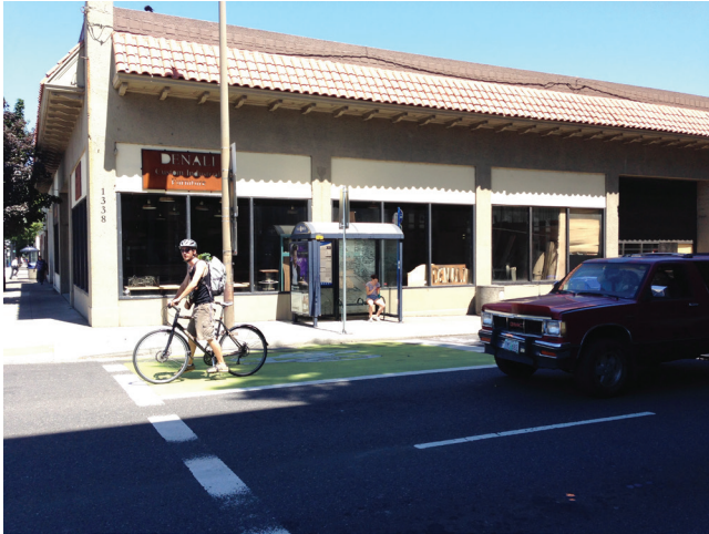
FIGURE 31 Green bike box at an intersection.
