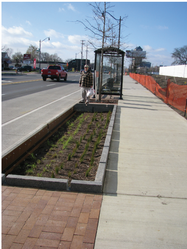
FIGURE 18 Rain garden blocking exit path from rear door of bus.
