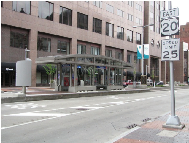
FIGURE 13 BRT bus station on left side of street in downtown Cleveland.
