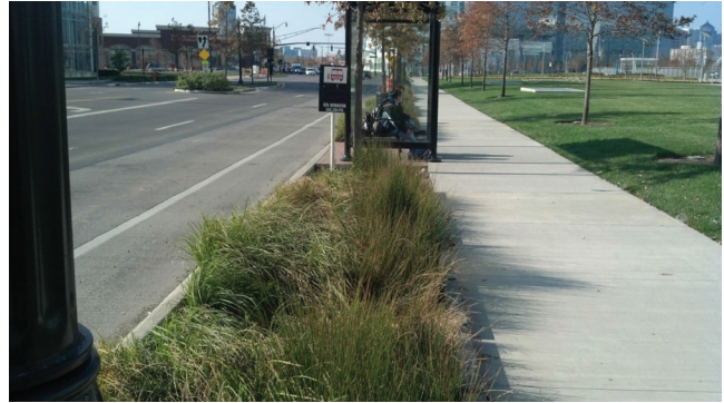
FIGURE 23 Rain garden improperly installed at bus stop.
