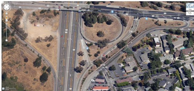
FIGURE 33 Golden Gate Transit freeway stop, Northbound US-101 and Tiburon Boulevard, Marin County.
