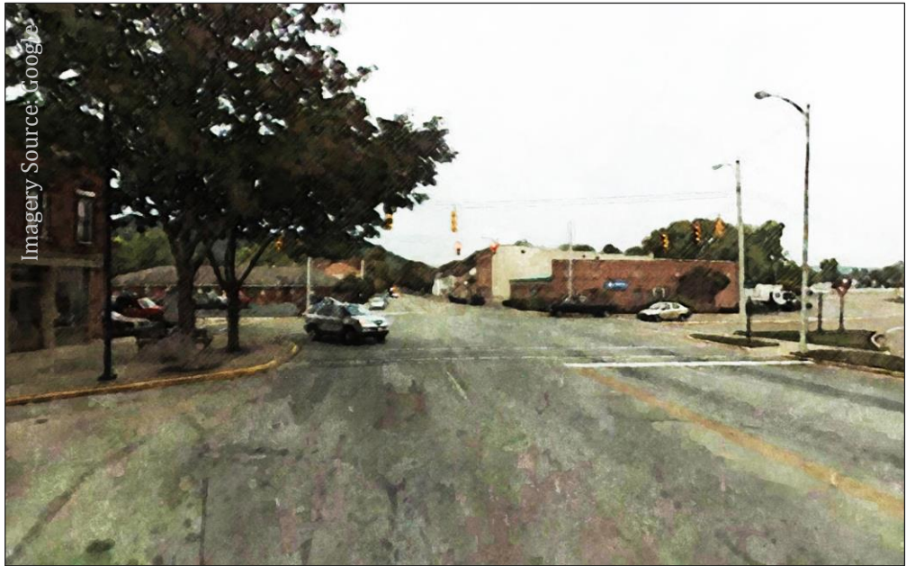
Figure 82 (above). View 2 of Water St., Chillicothe: Present.
