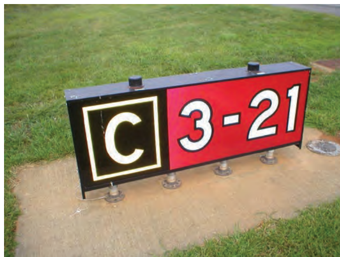
Figure 4.5. Well-maintained airfield sign. Source: Delta Airport Consultants, Inc.
