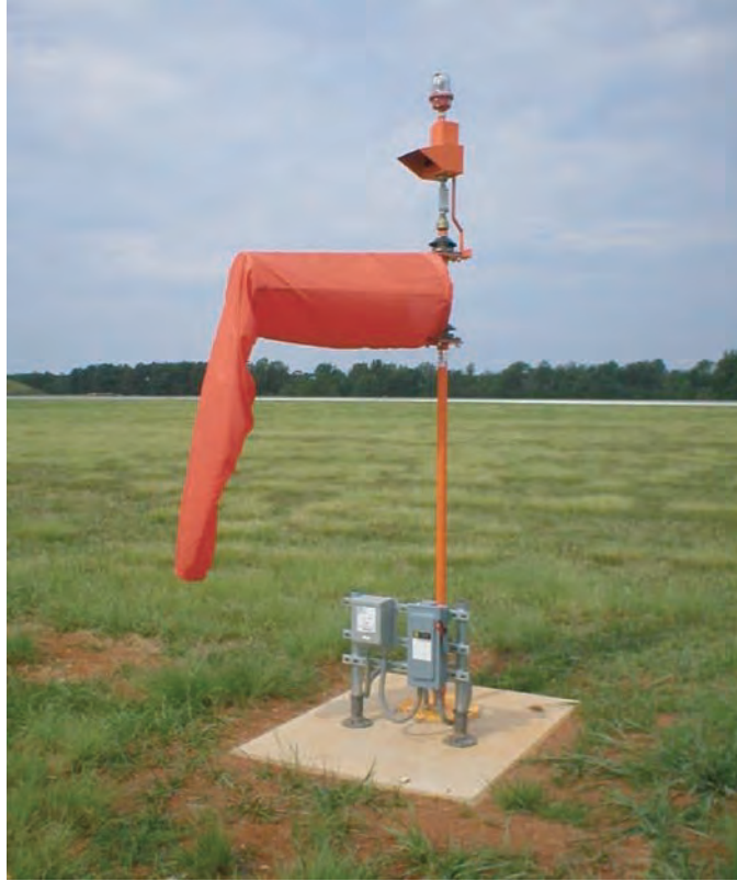
Figure 4.7. Wind sock. Source: Delta Airport Consultants, Inc.
