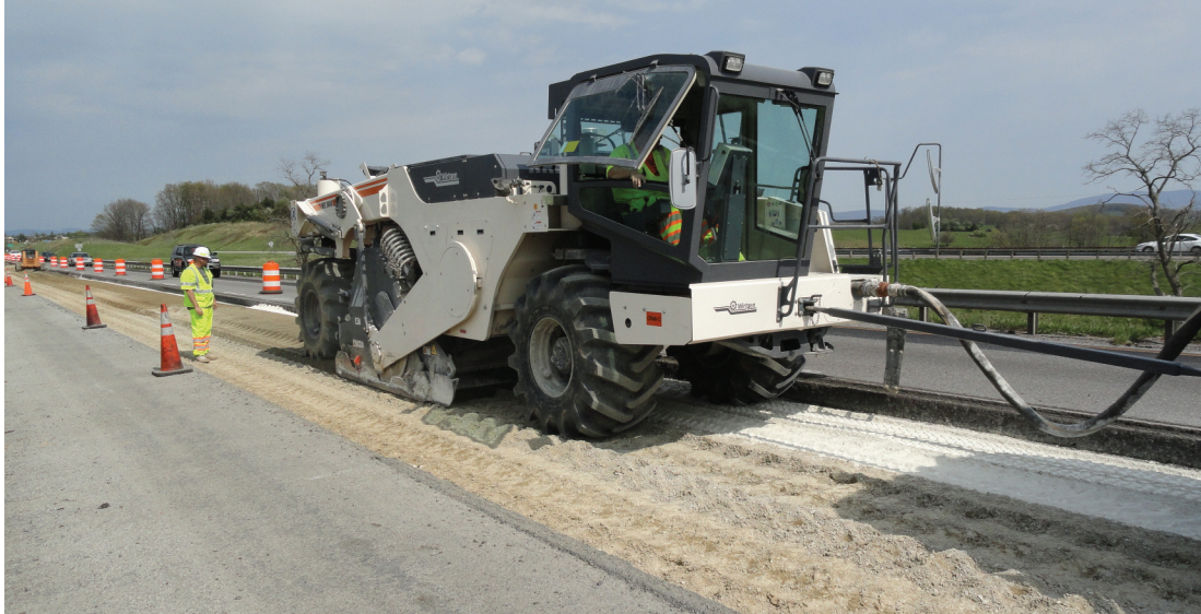
Full-depth reclamation on Interstate 81.
