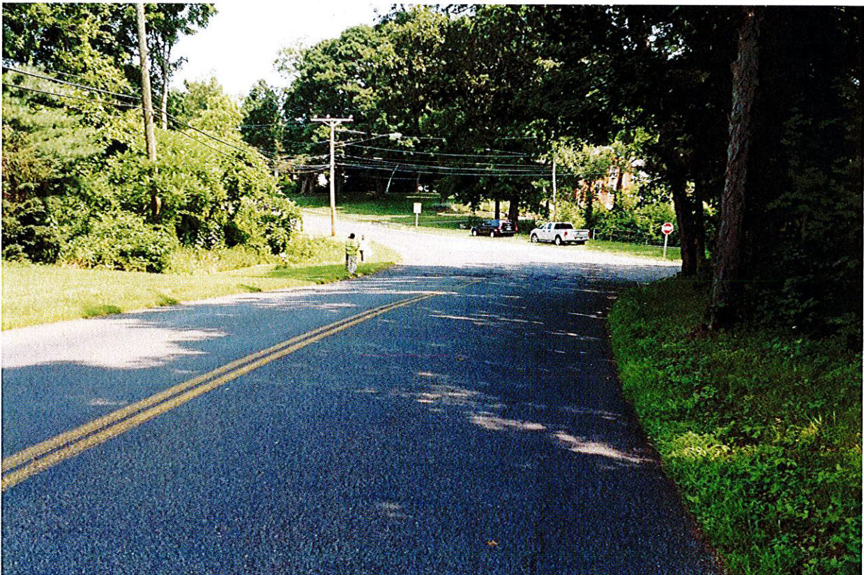
Graham Road northerly with RSA team members
