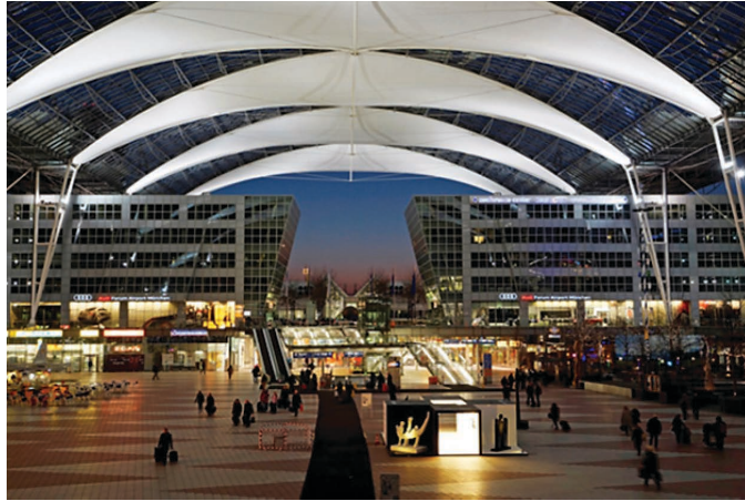
Figure A-7. Munich Airport Center.
