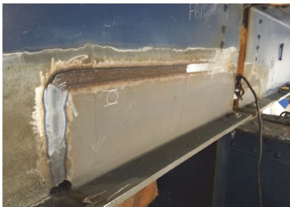
FIGURE 25 Massachusetts DOT stringer beam end repairs.
