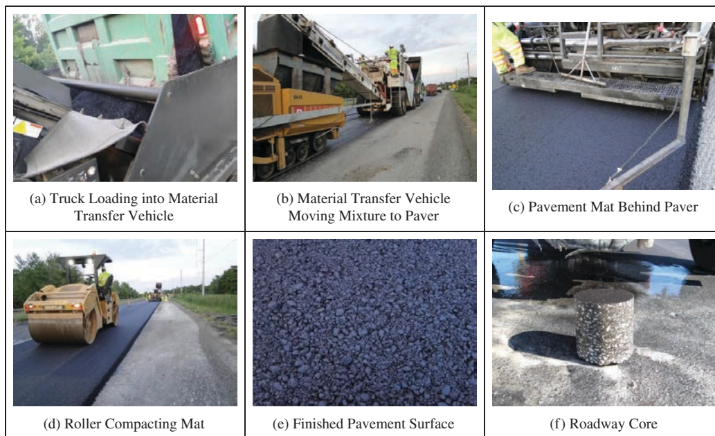
Figure 4-3. Plant-mixed-field-compacted (PF) specimen fabrication.
