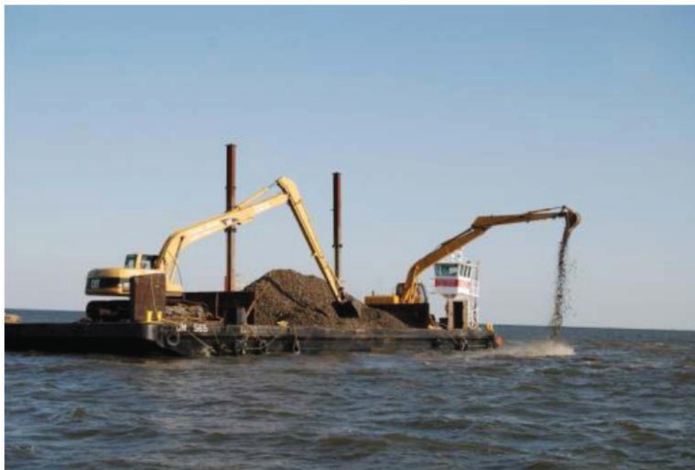
Figure 7.A Placing oyster reef shell as part of an oyster reef restoration and adaptive management project in Apalachicola Bay. SOURCE: Alabama Marine Resources Division.
