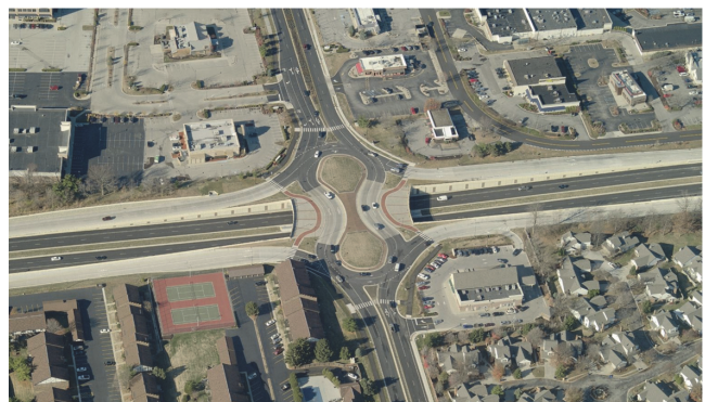
FIGURE 13 Keystone Parkway/E 116th Street intersection in Carmel, Indiana. Source: Microsoft Corporation (13).
