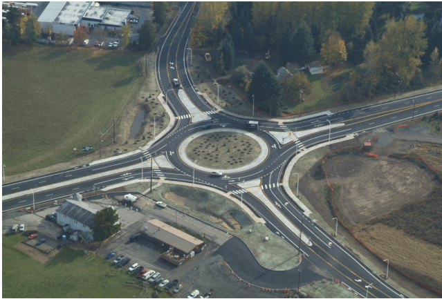
FIGURE 9 Multilane roundabout, SW Stafford Road/SW Borland Road intersection in Tualatin, Oregon. Source: Kittelson & Associates, Inc. (9).
