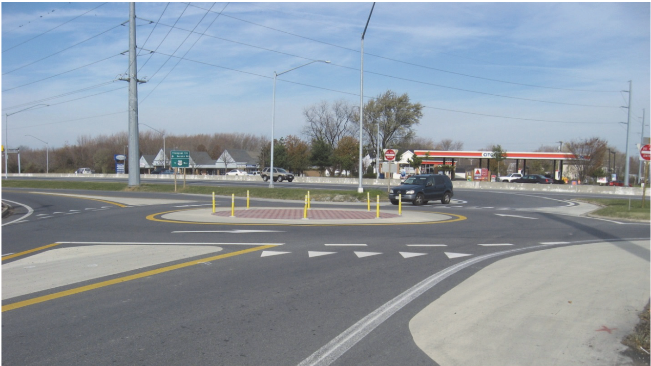
FIGURE 37 Accelerated low-cost roundabout installation at the intersection of US-50/Thompson Creek in Stevensville, Maryland. Source: Jenior (51).
