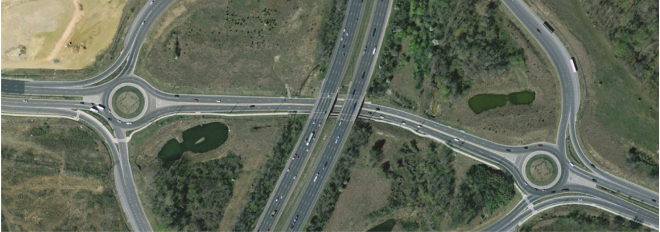
FIGURE 31 As-constructed I-495/Ritchie-Marlboro Road ramp terminal roundabouts. Source: Google Earth Aerial (48).
