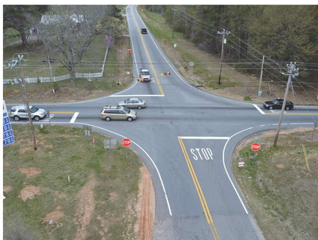
FIGURE 33 Intersection of SR-11/SR-124/Galilee Church Road in Jackson County, Georgia, prior to construction. Source: Zehngraff (50).
