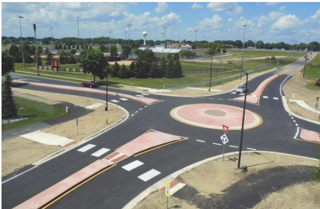
FIGURE 7 Mini-roundabout, Vierling Drive/County Road 79 intersection in Shakopee, Minnesota. Source: City of Shakopee (7).
