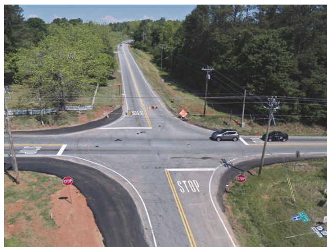
FIGURE 34 Intersection of SR-11/SR-124/Galilee Church Road in Jackson County, Georgia, during first weekend of construction of the accelerated low-cost roundabout. Source: Zehngraff (50).
