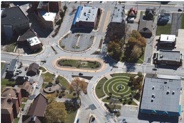
FIGURE 10 Rochester roundabout, Brighton Avenue/Adams Street (SR-68)/Rhode Island Avenue (SR-18) intersection in Rochester Borough, Pennsylvania. Source: Whitman Requardt & Associates, LLP (10).
