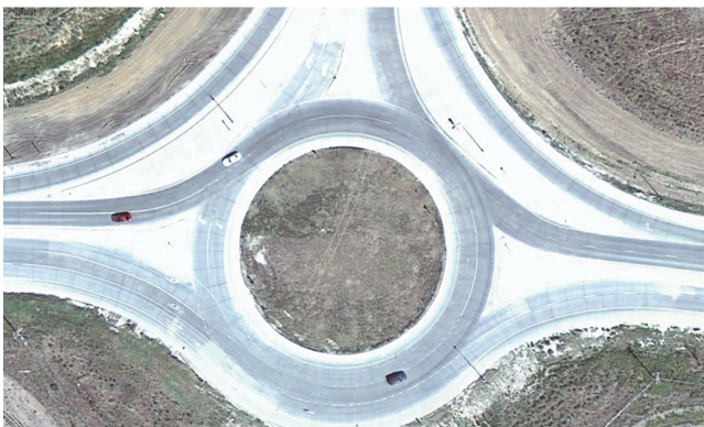
FIGURE 29 As-constructed US-50/Connector Road Roundabout in Emporia, Kansas. Source: Google Earth Aerial (46).
