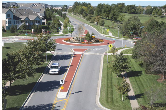
FIGURE 8 Single-lane roundabout, 133rd Street/Lamar Avenue intersection in Overland Park, Kansas. Source: City of Overland Park, Kansas (8).
