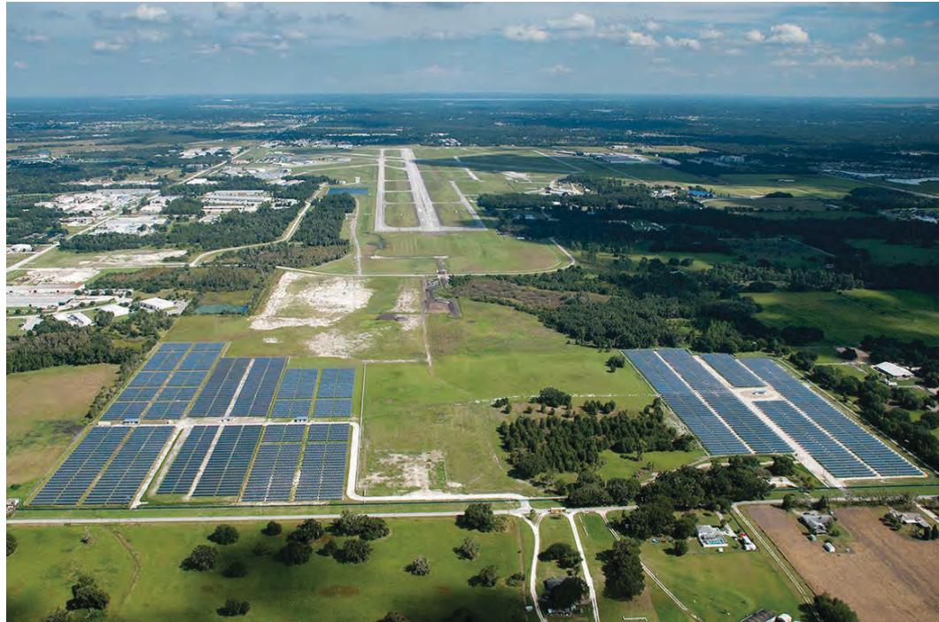
FIGURE 9 Lakeland Linder Regional Airport PV solar field (Source: B. Fay 2014).
