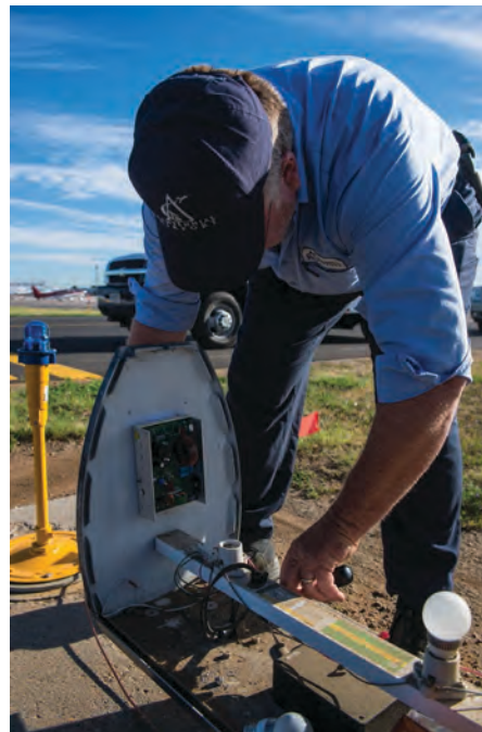
FIGURE 8 LED signage lighting retrofit (Source: L. Hinton 2015).
