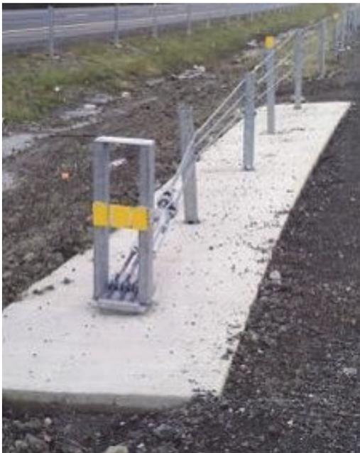
the clear zone. The end anchor consists of an in-ground anchor post, a cable release post and four terminal posts. The end terminal section is 27.5' in length. End anchors should be installed in AASHTO standard soils and be well drained. If soils do not meet these criteria, then soil testing should be done by the DOT or contractor, as per the state's specifications.
