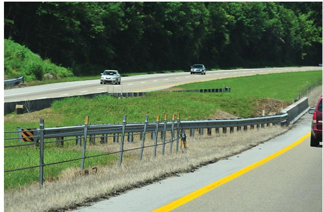
FIGURE 14 HTCB terminated in front of w-beam.
