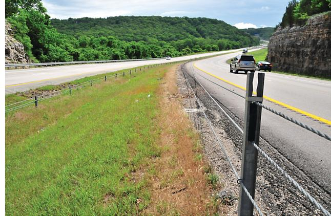
FIGURE 5 Impacted cable on outside of curve.
