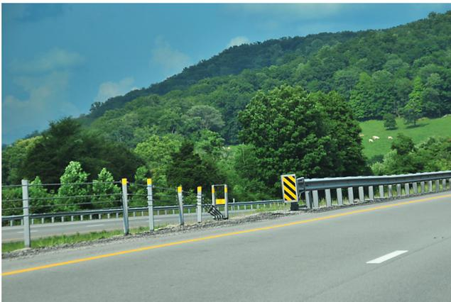
FIGURE 9 Terminating the HTCBB in advance of w-beam.
