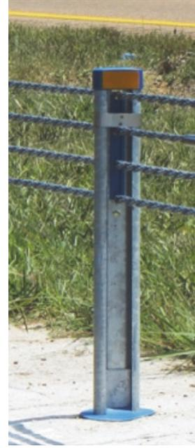
The system configurations using the C-post with a vertical slot at the top of the post are shown below. The direct driven option is shown, but a socketed post design is also available with a 450 mm (17.7 in.) socket and 1230 mm (48 in.) long C-Posts.
