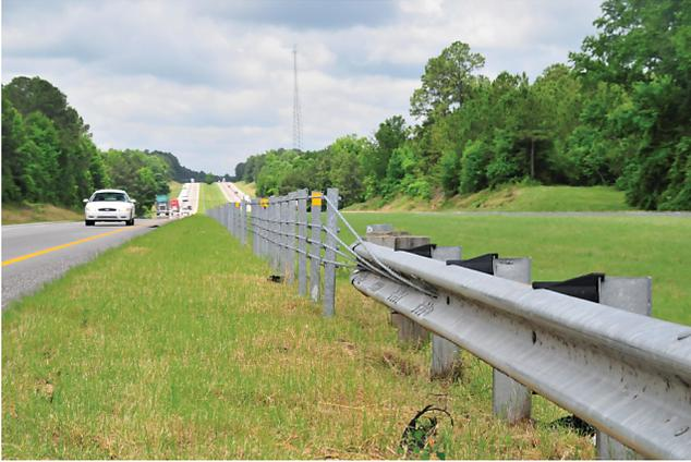
FIGURE 11 HTCB connected directly to w-beam.
