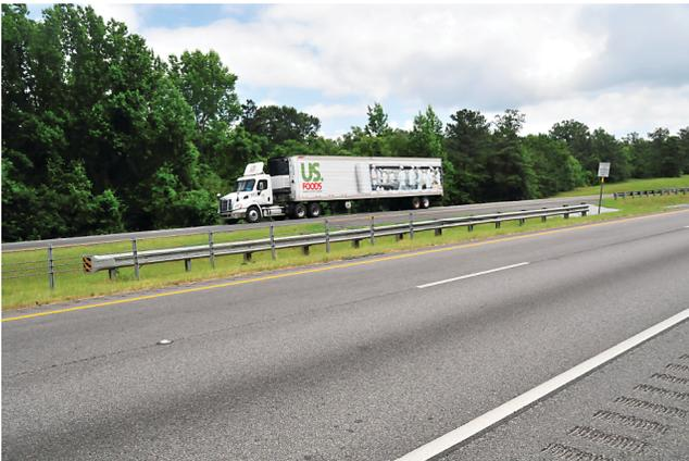
FIGURE 12 Short section of w-beam installed as an “anchor.”
