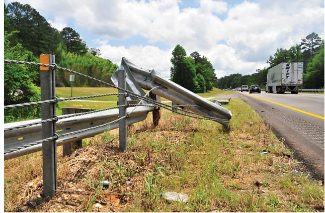
FIGURE 13 Inadequacy of HTCB connection to short run of w-beam.
