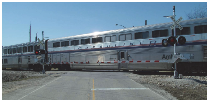
Figure 5-1. Four-quadrant gate installation on intercity passenger rail line.
