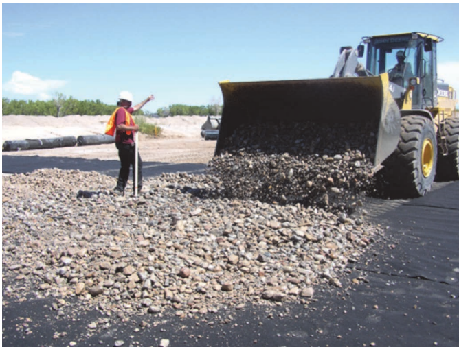
Figure 4.40. Granular filter placement over geotextile fabric.
