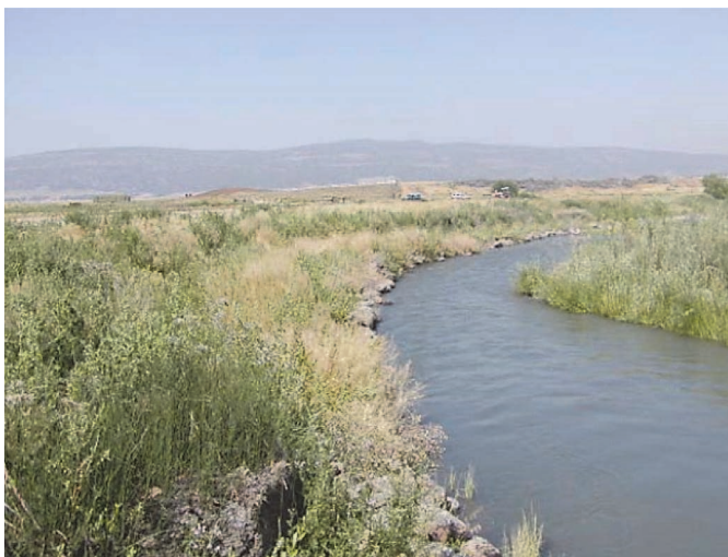
Figure 4.24. Revegetation of eroding bank landward of stone toe (photo by J. McCullah).
