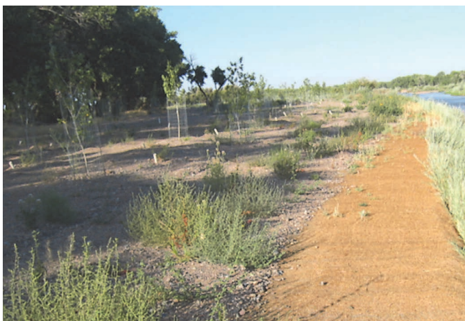
Figure 4.43. View of willow-planted FES bankline and planted willow poles in overbank area.
