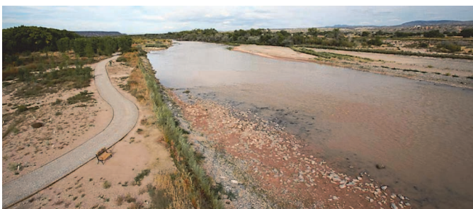
Figure 4.45. View looking upstream of upstream end of GRF #3 with vegetated FES along right bank, planted willow poles and vegetation in right overbank area, and left bank transition guide bank with planted willows.
