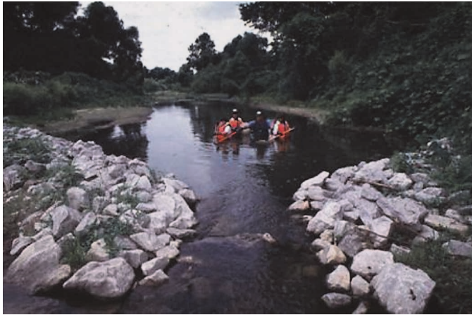
Figure 4.17. Weirs can create pool-riffle habitats and help stabilize beds, but should be designed carefully in streams with low bed slope to prevent eliminating current during low flow (McCullah and Gray 2005).
