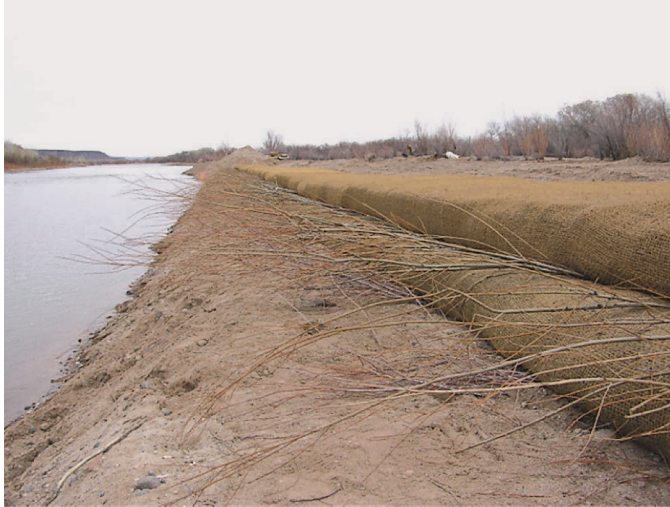
Figure 4.42. View of FES and willow plantings immediately after installation.
