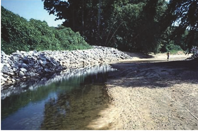
Figure 4.16. Stone toe provides stable benthic habitat and cover for smaller fish, but little diversity or pool habitat (McCullah and Gray 2005).
