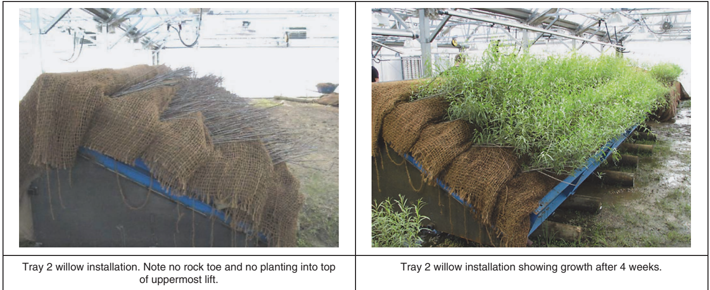
Figure 3.6. Tray 2 installation.
