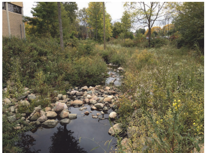
d. Stone cross vane two years after construction.
