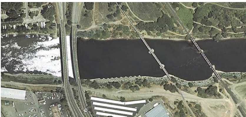
Figure 2.9. 2002 aerial photo of LAR reach RM 2.0L.
