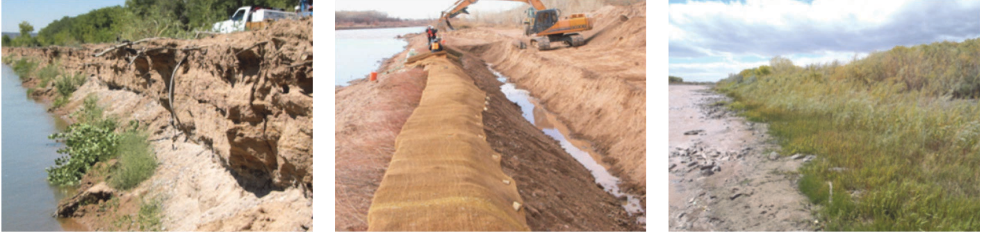
Figure 4.44. Before, during, and after views of willow-planted FES over rock riprap at GRF #3.
