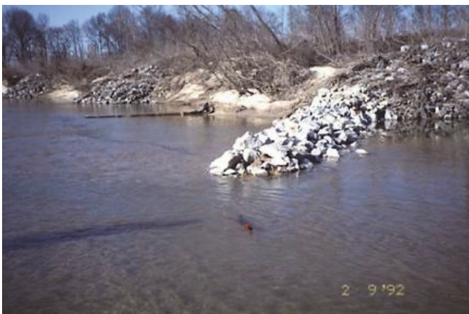
Figure 4.18. Spurs, barbs, and bendway weirs provide local zones of low velocity that are effective refuges (McCullah and Gray 2005).
