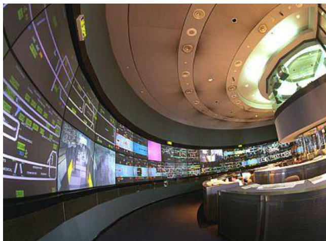
FIGURE 22 MBTA operations control center. Source: MBTA.
