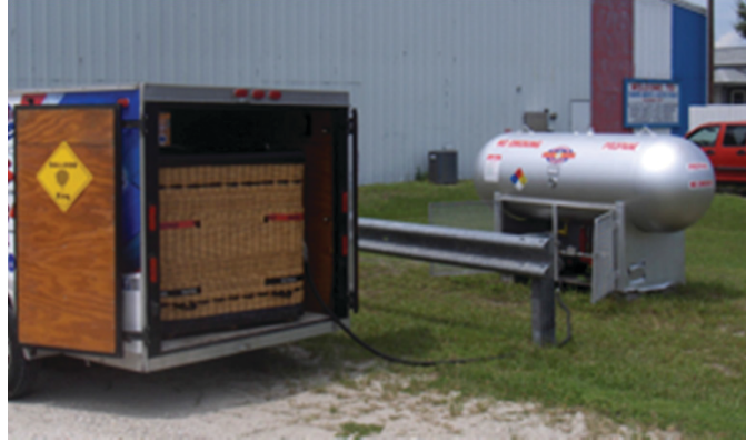
FIGURE 8 Propane storage tank located at an airport (Credit: S. Quilty, SMQ Airport Services, Lutz, Florida. Used with permission.).
