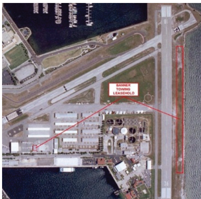
FIGURE 47 Banner towing operational lease areas contained in a request for proposal (Source: R. Lesniak, Albert Whitted Airport, Florida. Used with permission.).
