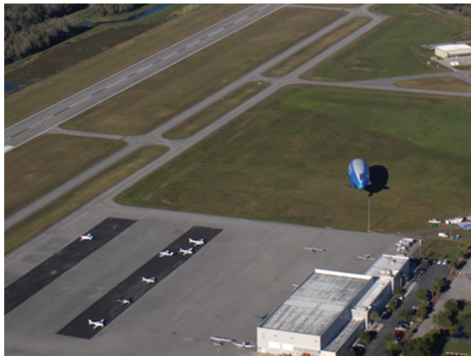
FIGURE 9 Blimp positioned and moored away from aircraft movement areas ( Credit: S. Quilty, SMQ Airport Services, Lutz, Florida. Used with permission. )
