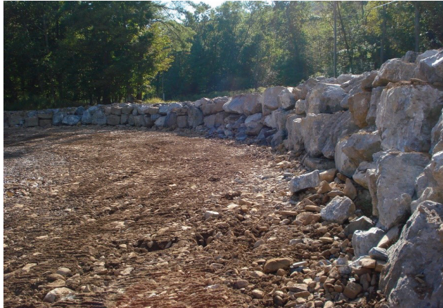
FIGURE 48 Repairing bank with riprap (Courtesy of WVDOT).
