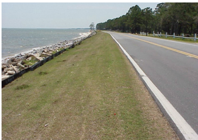
FIGURE 18 Roadway after completion of repair work (Courtesy of Florida DOT).
