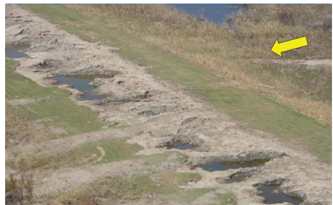
FIGURE 95 Overtopped earth embankment totally eroded by 2 hours of hurricane surge overtopping (Briaud 2008).
