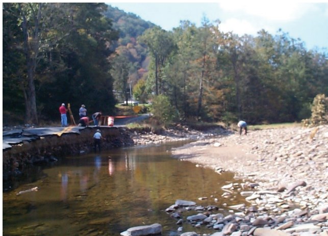
FIGURE 44 Slope erosion and pavement undermining after Hurricane Isabel in 2003 (Courtesy of WVDOT).
