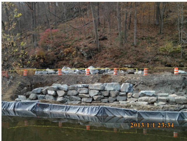
FIGURE 41 Implicated stone wall under construction (Courtesy of Maryland DOT).
