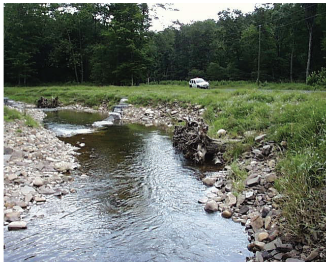
FIGURE 46 Channel reconstruction after Hurricane Isabel in 2003 (Courtesy of WVDOT).
