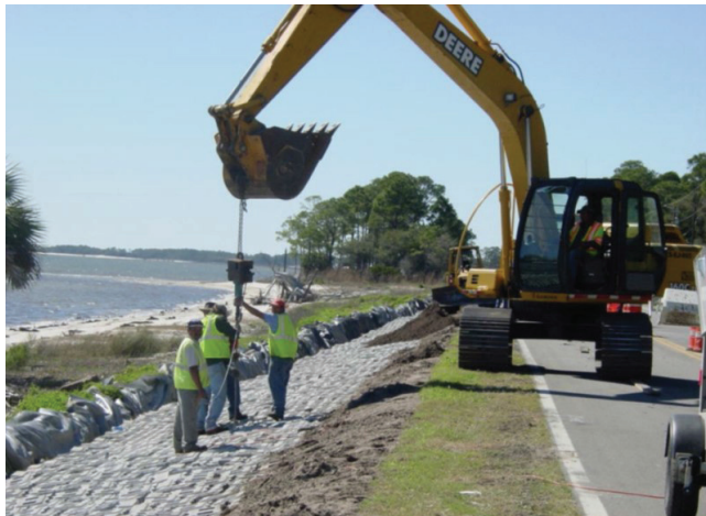
FIGURE 17 Construction of stabilized roadway section (Courtesy of Florida DOT).
