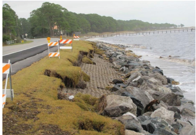
FIGURE 19 Damage limited to the removal of performance turf and topsoil after armoring (Courtesy of Florida DOT).
