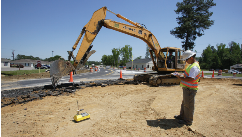
PHOTO: AL COVER, VIRGINIA DOT
