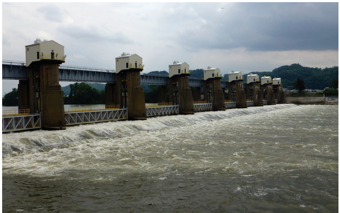
Emsworth Locks and Dams on the Ohio River, U.S. Army Corps of Engineers Pittsburgh District.
