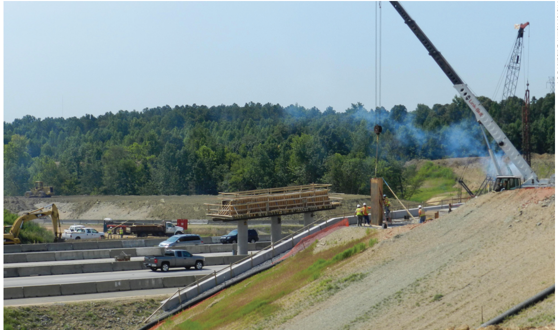
PHOTO: NORTH CAROLINA DOT
