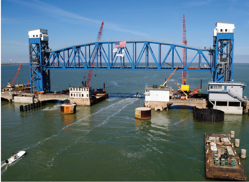
A new Galveston Causeway Railroad lift bridge over the Gulf Intracoastal Waterway allowed widening of the navigation channel through the draw span.
