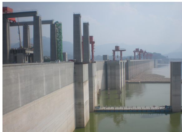
FIGURE 1.2.1 Three Gorges Dam. SOURCE: Courtesy of Keith Clarke, University of California, Santa Barbara.
