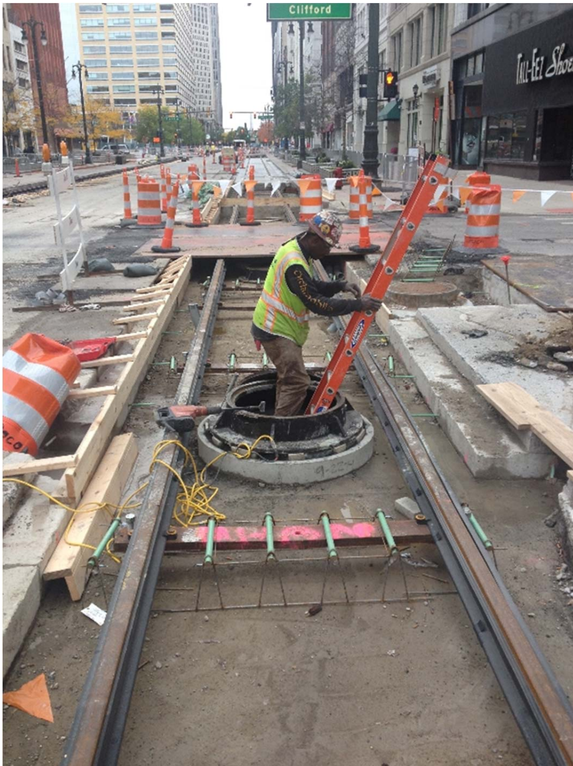
FIGURE 9 Construction of the M-1 RAIL streetcar required reconstruction of streets that had 300 years of utilities and other infrastructure beneath them.
