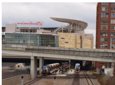
Metro Transit, Minneapolis, MN
