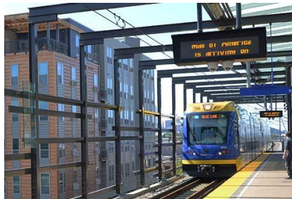
Metro Transit, Minneapolis, MN
