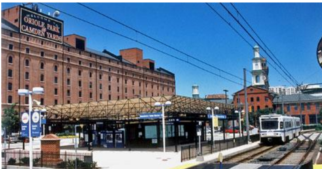
FIGURE 2 MTA Camden Yards Station.
