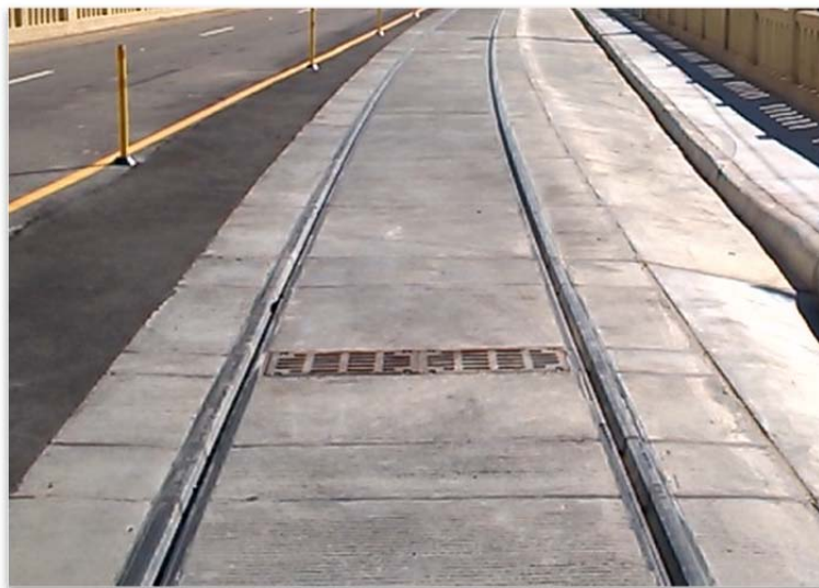
FIGURE 5 112TRAM embedded track: Dallas.
