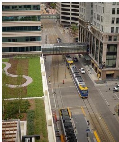
Metro Transit, Minneapolis, MN
