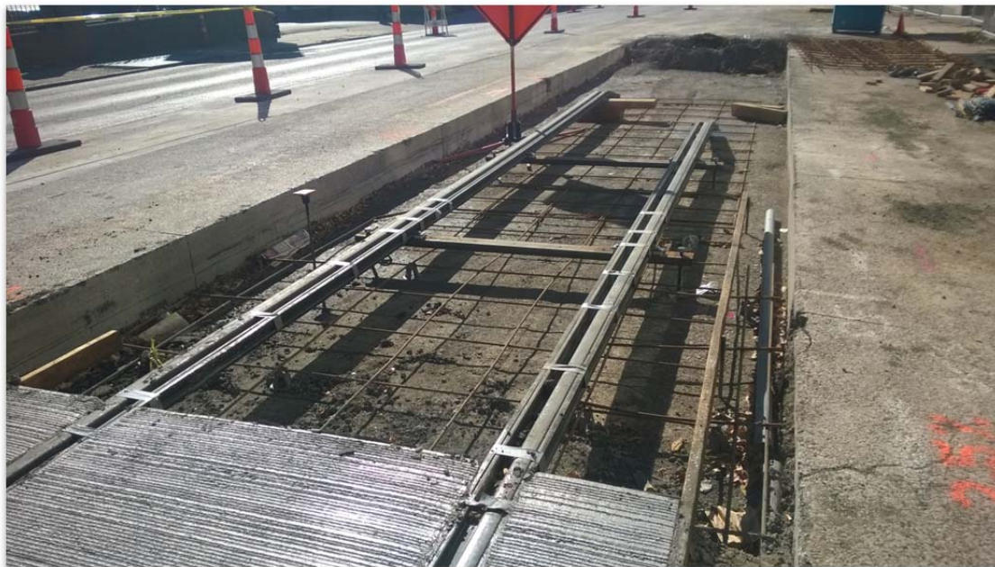
FIGURE 6 112TRAM installation: Kansas City.
