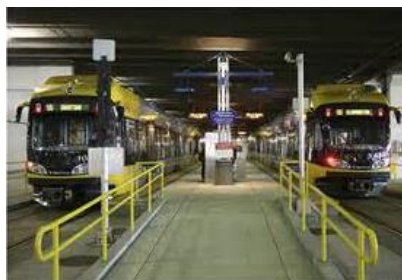
Maintenance Facility, Metro Transit, Minneapolis, MN
