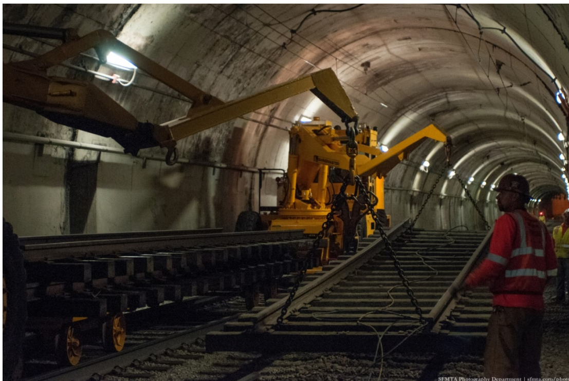
FIGURE 10 Sunset Tunnel construction.
