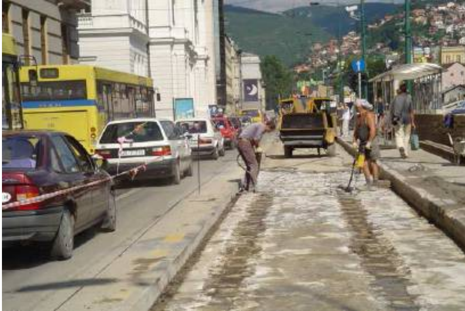
FIGURE 8 Works in modernization of tramway tracks in Sarajevo.
