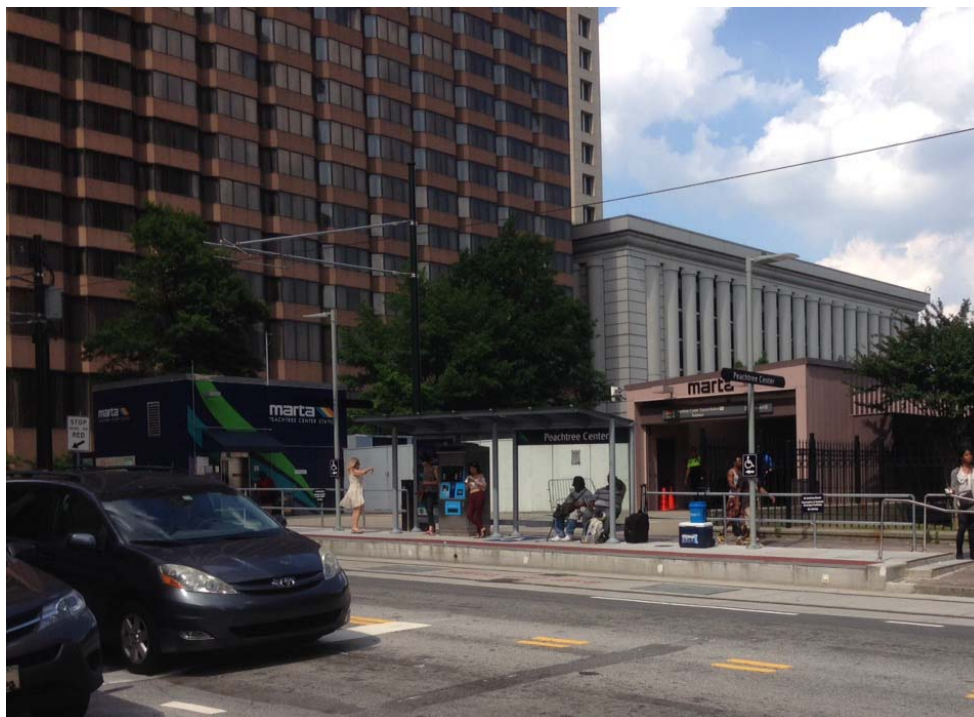
FIGURE 1 The Atlanta Streetcar stop is immediately outside the portal to the MARTA Peachtree Center Station.
