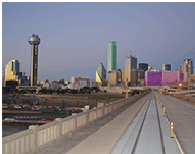
FIGURE 1 Dallas Streetcar Houston Street Viaduct Bridge (looking north).
