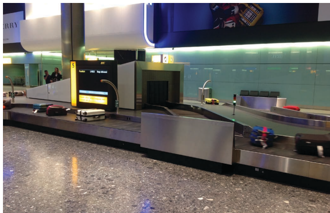
Figure 4-30. Remote-fed flat-plate baggage claim carousel at Heathrow Airport Terminal 2.
