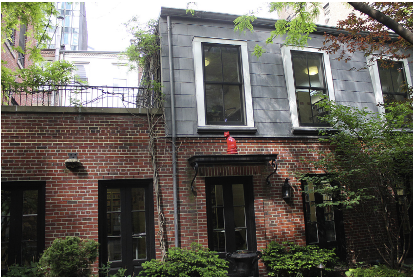
Library seen from the courtyard.
