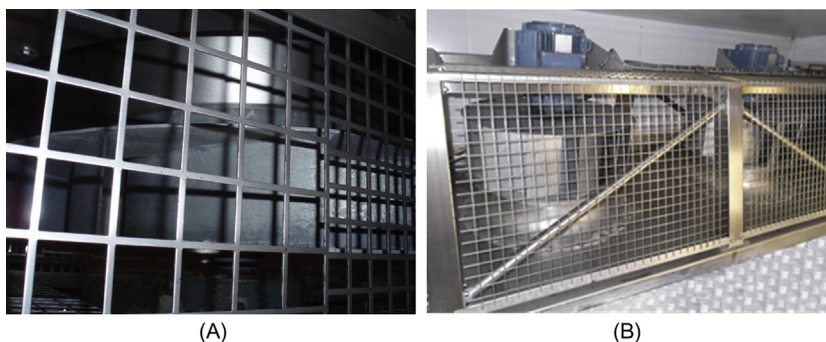
FIGURE 6.60 Stainless steel guards: (A) Punched sheet (>95% open) gives good protection against the centrifugal fan, while allowing access for cleaning and disinfection. (B) Weld mesh guards positioned around the centrifugal fans have a sloped top surface. The fans themselves are positioned inclined on a sloped surface, allowing maximum drainage of condensate and cleaning liquids to the front side.
