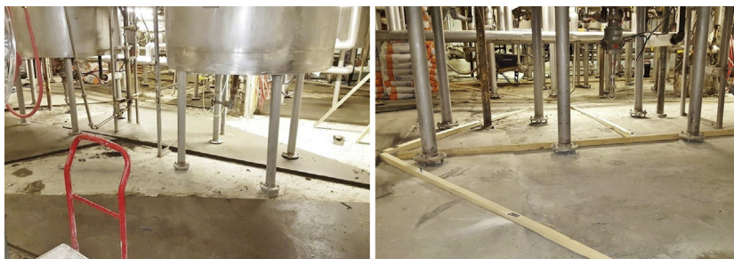
FIGURE 6.23 By anchoring the process equipment to the floor, it cannot move from its designated position during operation. Foot anchors should be polymer sealed into the floor. Grouting foot anchors into a concrete floor may give rise to unhygienic conditions with time. Courtesy of Surface Solutions, Inc.
