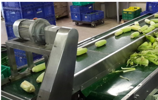
FIGURE 6.11 This motor without drip pan is positioned above the product stream, increasing the risk of lubricant dripping onto the food product. Dirt also may build up in the chain guard.
