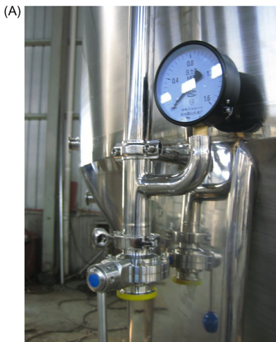
FIGURE 7.81 Pressure measurement devices installed on a too-long instrument branch.
