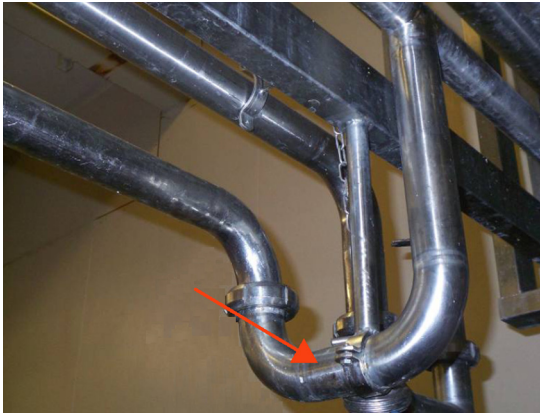
FIGURE 7.28 Nondrainable pipe section. Courtesy of Mondelez International, © 2016.
