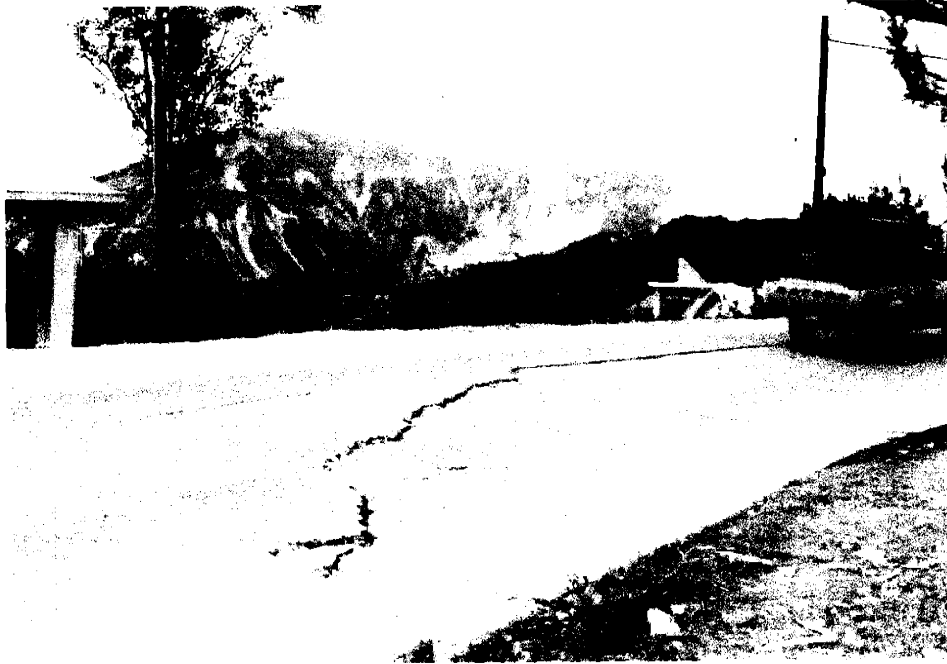
Figure 3.14 Effects of the 16 July 1990 Earthquake (Geotecnica, 1990)
