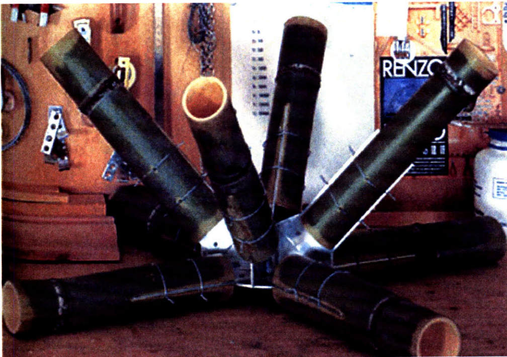
Figure 5-26 Bamboo-steel connection 39
