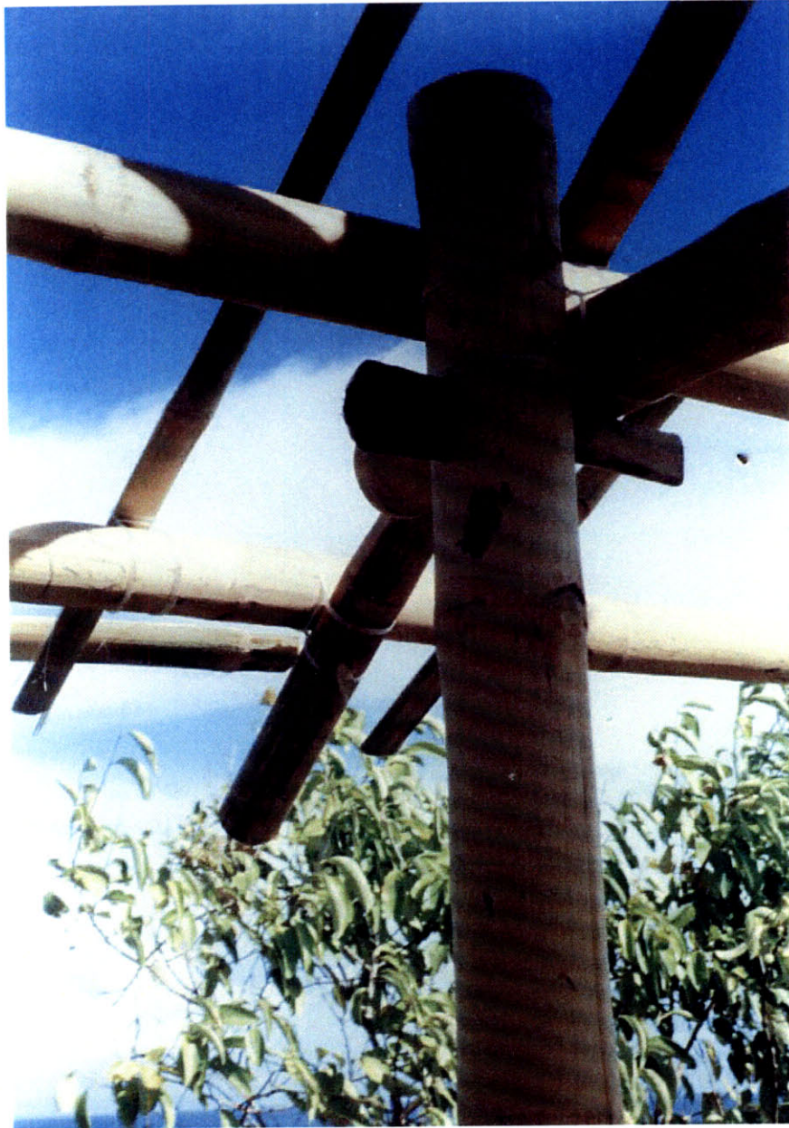
Figure 5-28 Beam-Column connection with lashing and dowel 41
