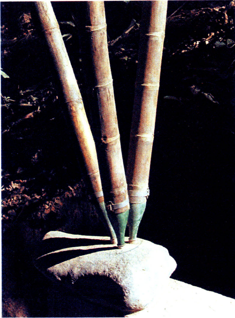
Figure 5-24 Other example of concrete-bottle-bamboo foundation
