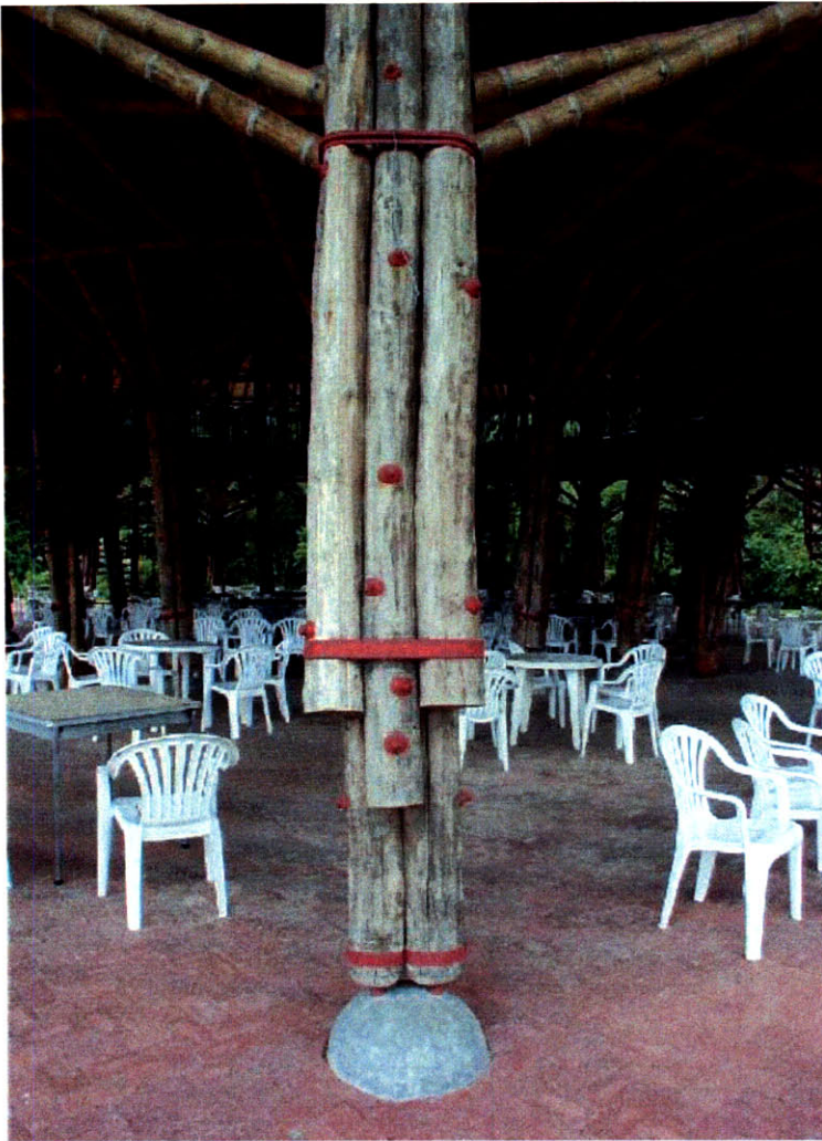
Figure 5-19 Compound Column in Simon Velez's ZERI Pavilion 37
