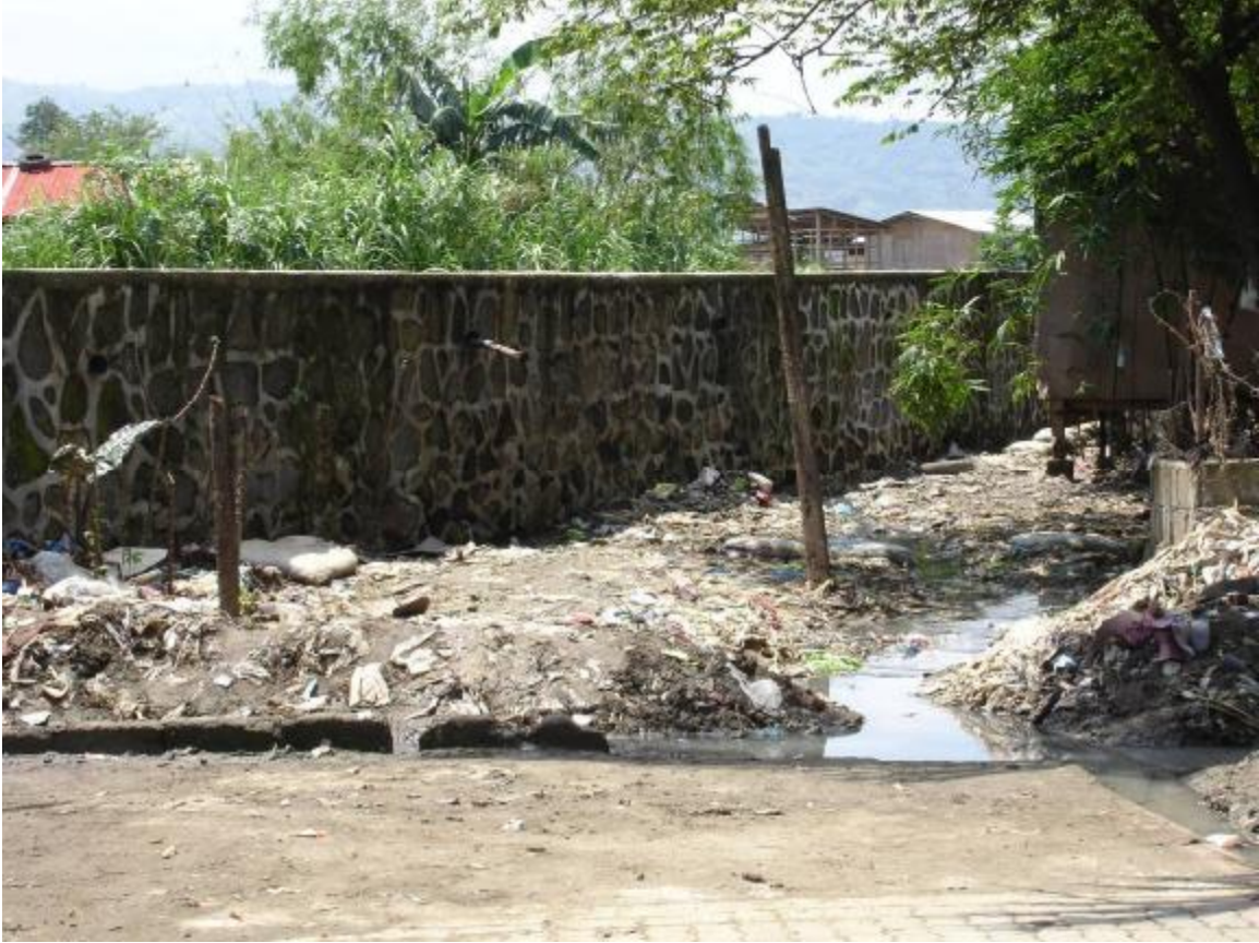
Figure 13 - GK Brookside (Manila). Site runoff moves untreated into neighbors' lots.
