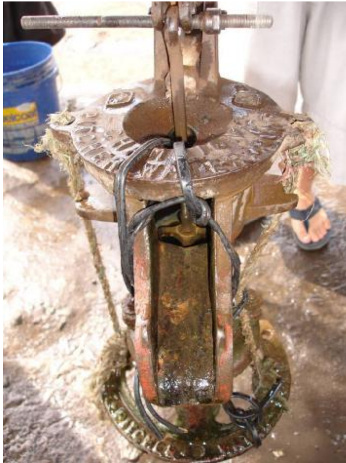
Figure 6 – GK First Calacan (Batangas). This well was growing algae and black slimy biomass.
