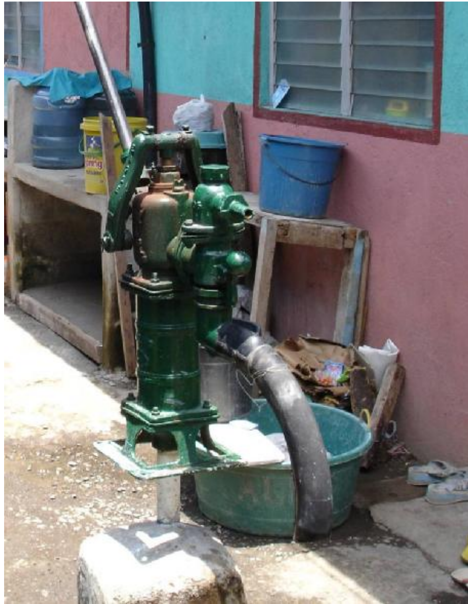
Figure 5 – GK San Francisco Javier (Batangas). Note the spout addition that can harbor bacteria.
