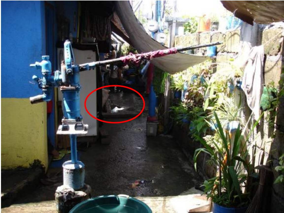
Figure 4 – GK San Francisco Javier (Batangas). Note the septic tank (circled in red) located too closely to the well.
