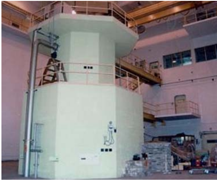
Figure 2.4 -TRIGA reactor and pool structure similar to the research reactor at Oregon State University. (This figure was obtained from Ref. 11 .)
