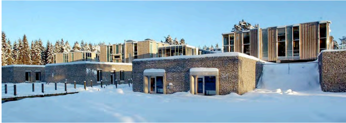
Figure 3.15. Exterior view of the school from the common courtyard.
