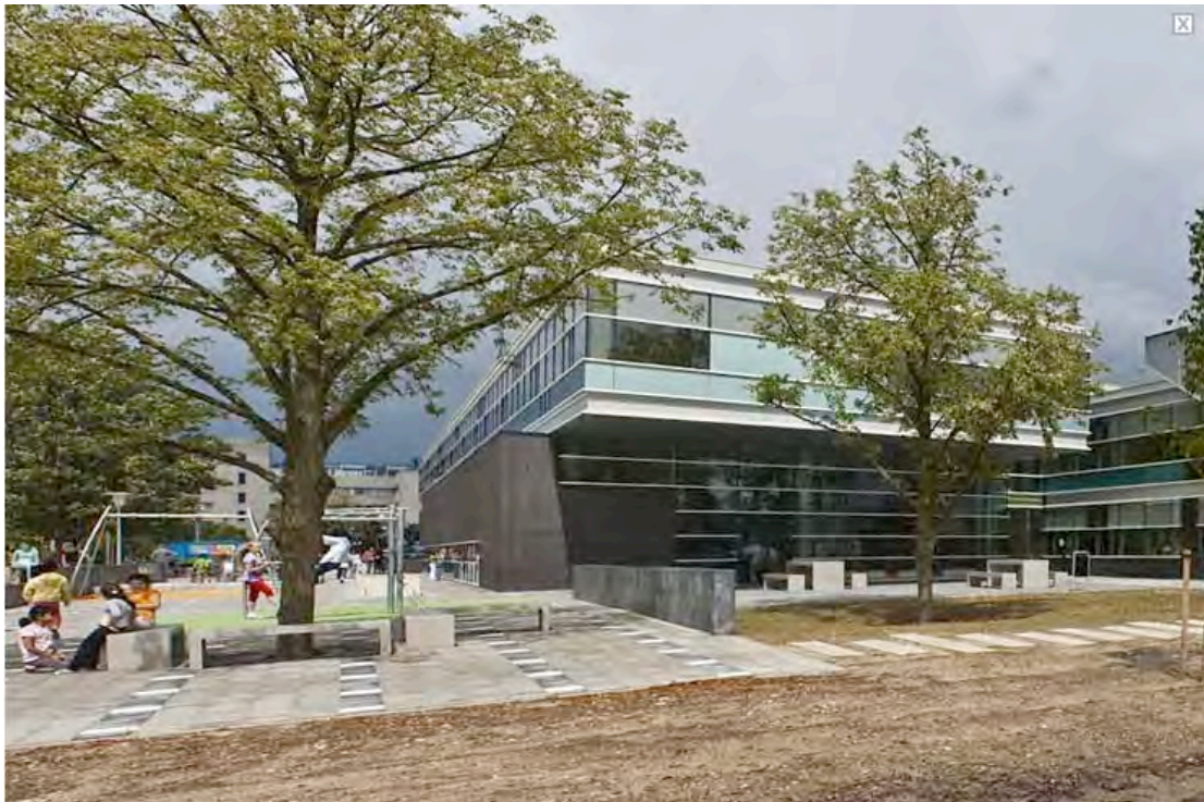
Figure 3.29. View of the building and of the school grounds.
