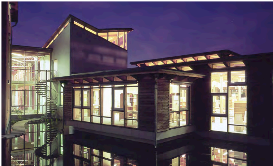
Figure 3.7. Nocturnal view of the ateliers.
