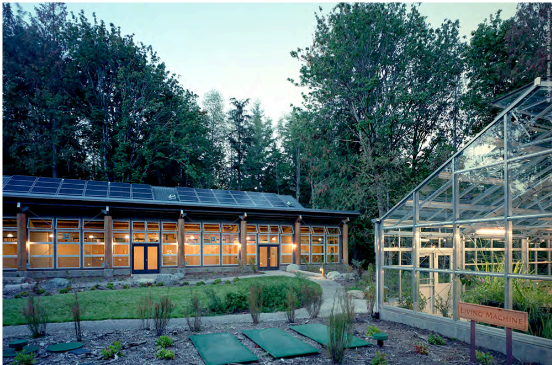
Figure 3.10. View of the learning studios and of the living machine.
