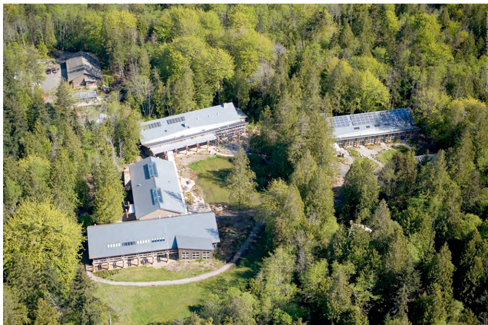
Figure 3.9. Aerial view of main buildings.
