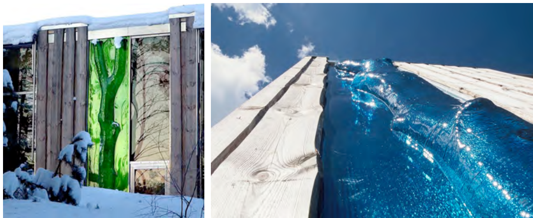
Figure 3.20. Logs are integrated into the exterior walls: reuse of onsite materials.
