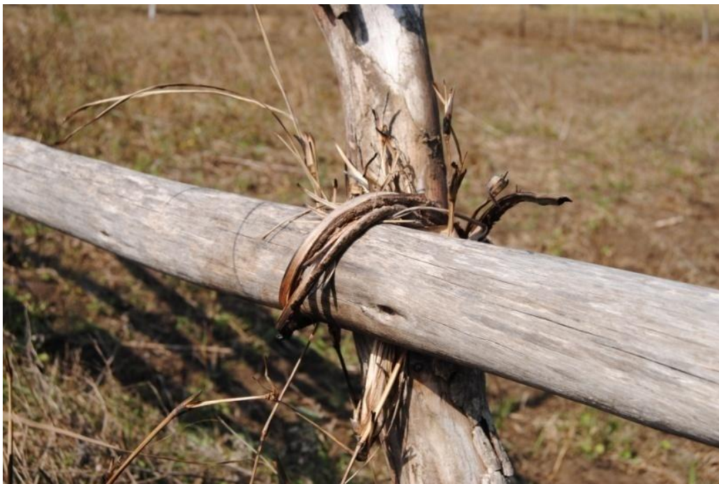
Figure 18. Detail of fence tie made of torn bark strips
