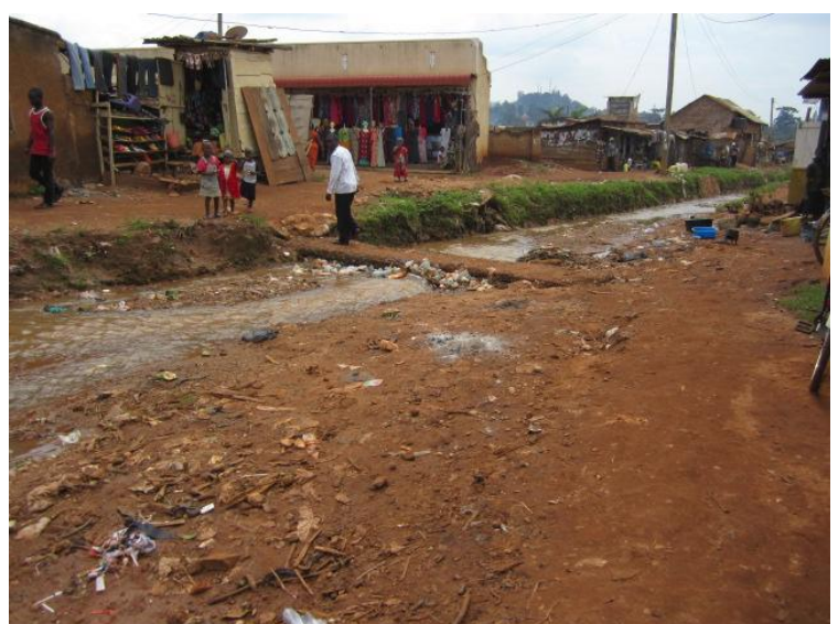
Figure 2. Blocked drainage channel in Bwaise Parish III. Photo:Solange Berleen Musoke, 2011
