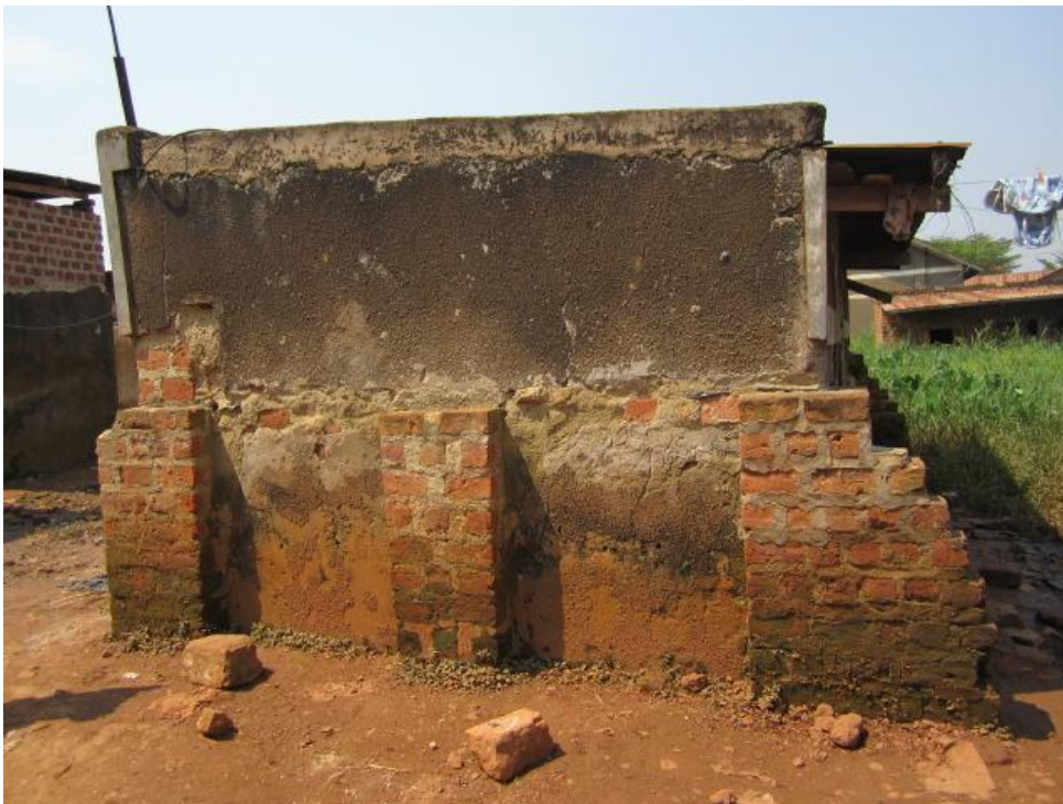
Figure 5. Unfinished exterior flood proofing of house. Photo: Solange Berleen Musoke, 2011
