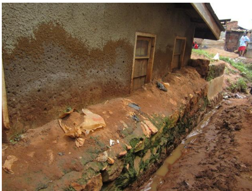
Figure 8. Flood proofed windows Photo: Solange Berleen Musoke, 2011
