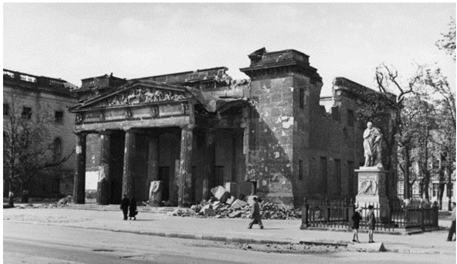
Fig. 28 Damaged exterior of Neue Wache, 1946.
