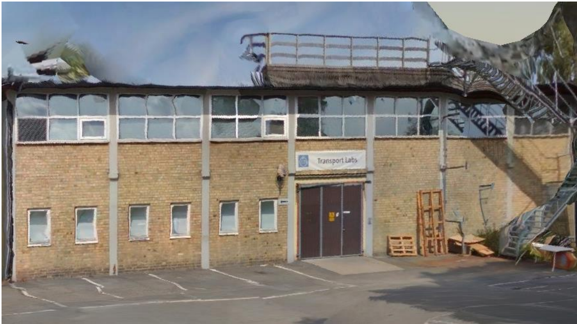
Figure 25 Screenshot in Smart3DCapture, building reconstructed from only street view images
