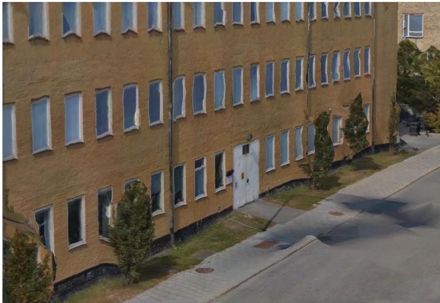
Figure 33 Screenshot in Smart3DCapture, façade reconstructed from street view images
