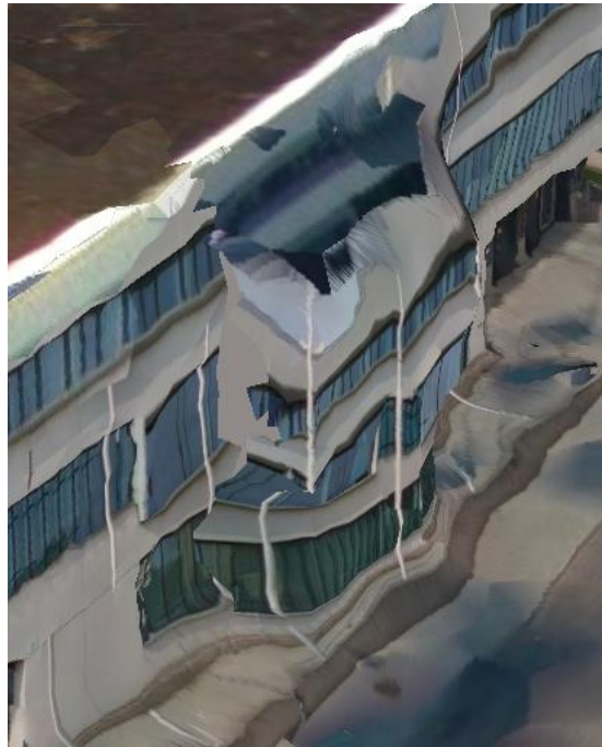
Figure 42 Screenshot in Smart3DCapture, flagpoles are destroying the building geometry
