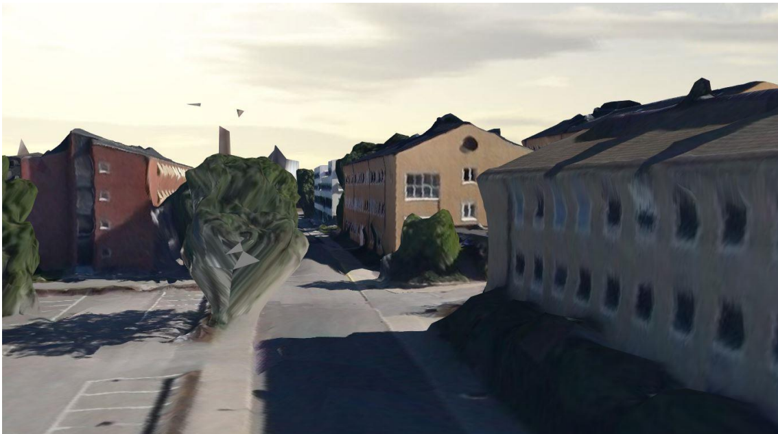
Figure 21 Screenshot in Smart3DCapture, street view of the model reconstructed from aerial images
