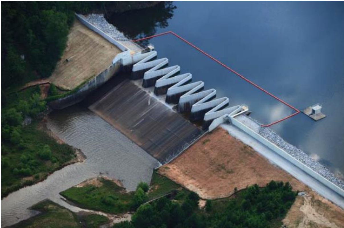
Figure 2.1 Raised labyrinth spillway, Dog River Dam, Georgia (U.S. Society on Dams, 2011)
