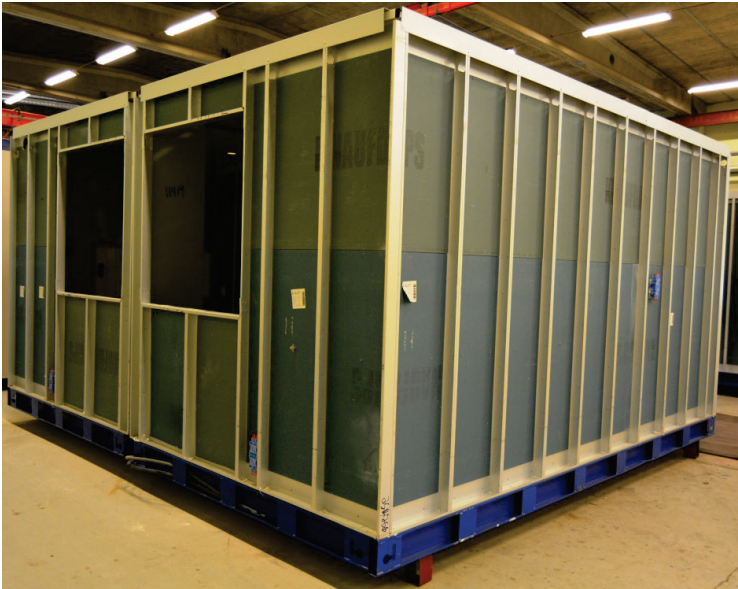
Figure A.7: Construction of 3D Module – 2 x 3D Modules together [27]
