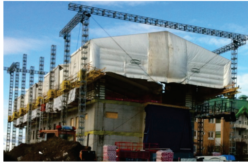
Figure 3.2: Overall protection of construction site (Sunderby hospital, 2014)
