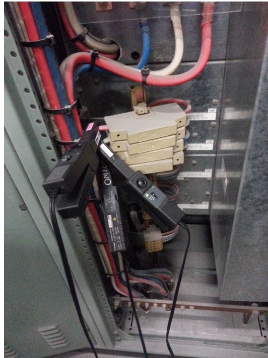
Figure 4.3: Data Sampling with the OMICRON CMC 256-Plus Using Analog Clamp-on's.
