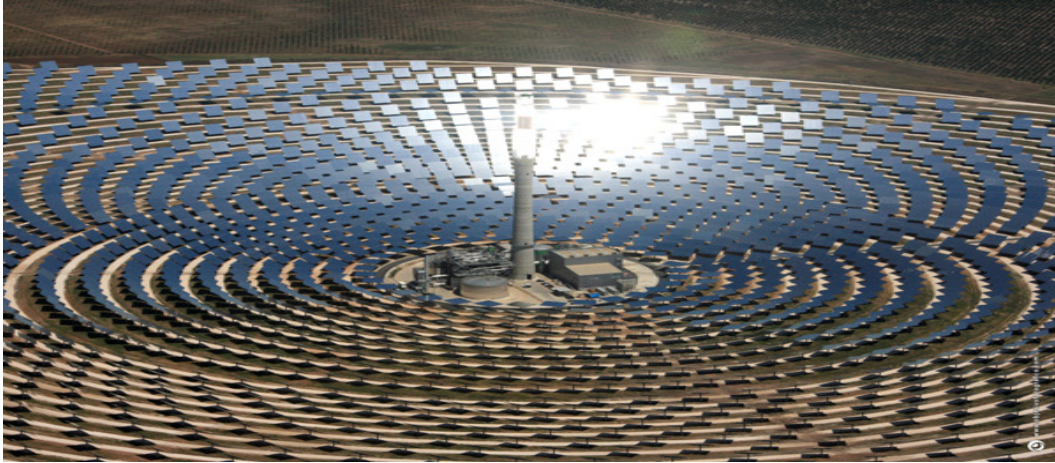
Figure 1.4: The heliostat field of a Central Receiver CSP plant. (Source: Wimberley, 2011).
