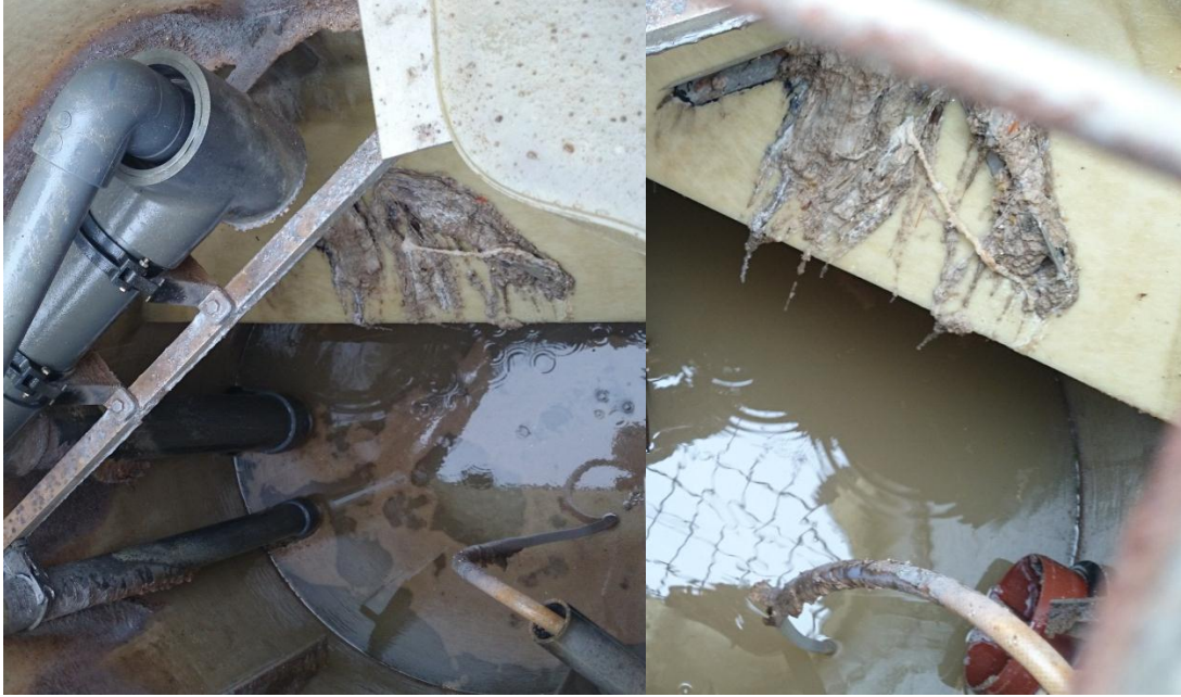
Figure 47. The cloth of organic material before installation of splash.
