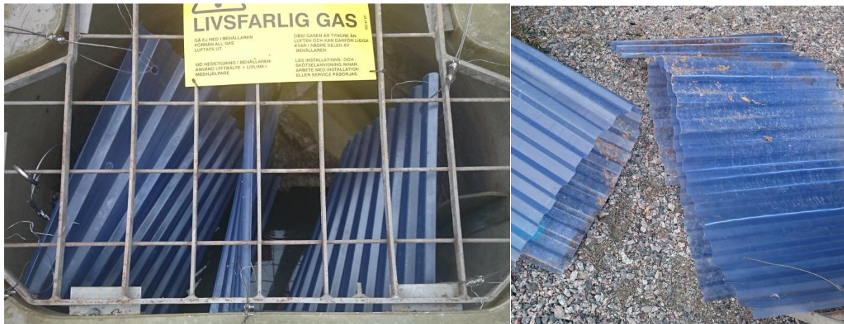
Figure 28. The plastic curtains hung inside Odomin.
