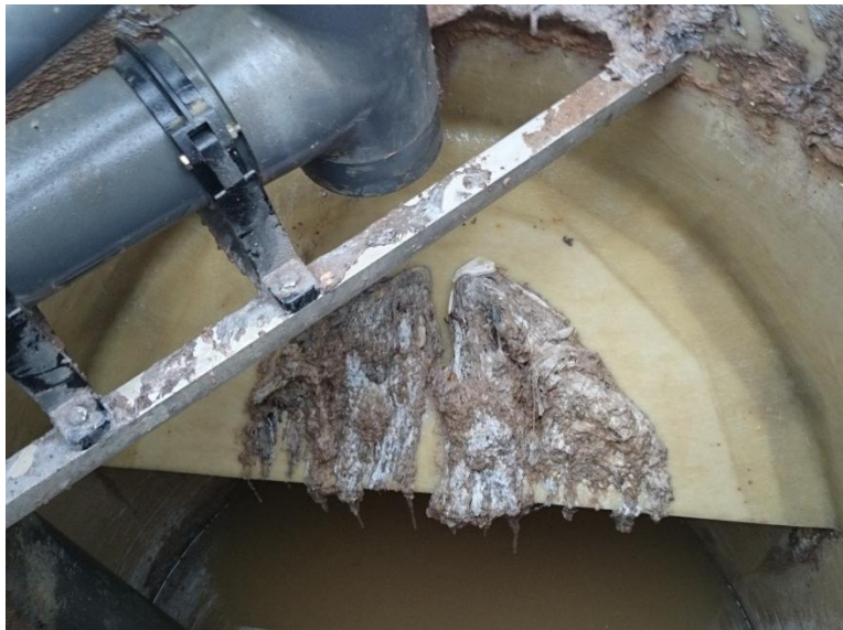
Figure 48. The cloth of organic material after installation of splash.
