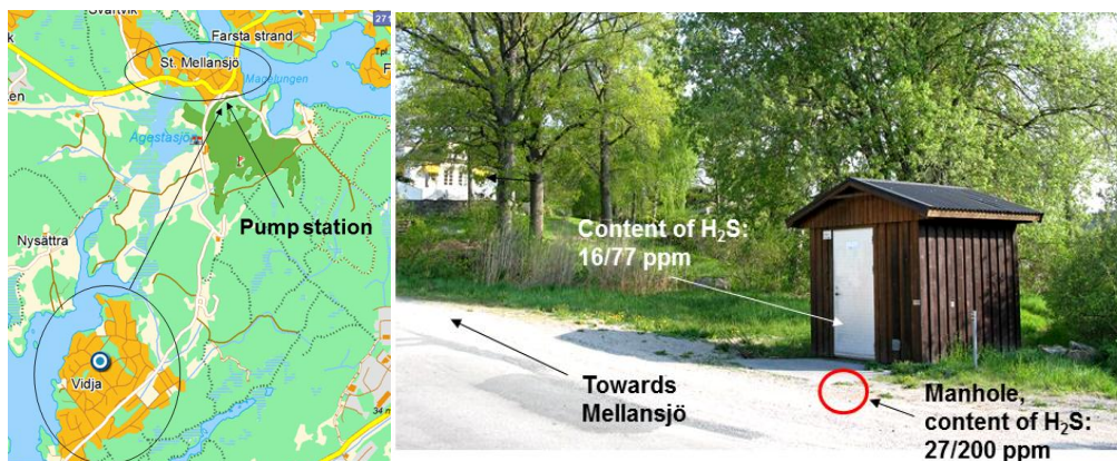
Figure 12. The pump station in Ågesta (Mellansjö).
