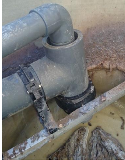
Figure 27. The splash mounted at the inlet in Odomin.
