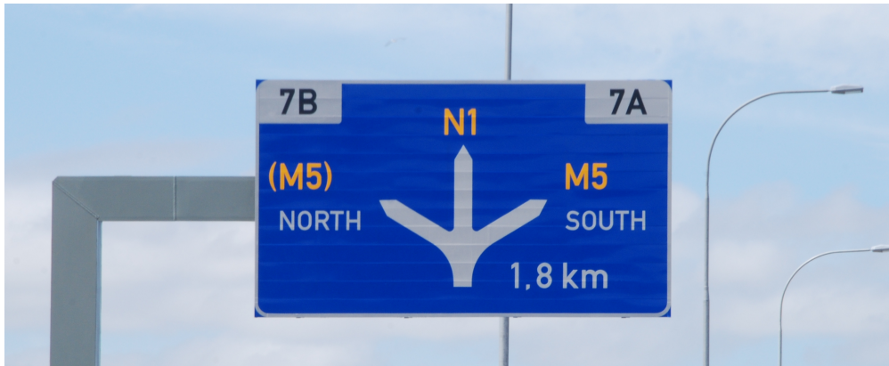
FIGURE 1.6: A guidance overhead freeway direction sign.
