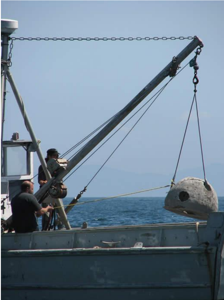
Figure 3. Photo of Reef Ball deployment method. A hydraulic davit on a landing craft was used to lower Reef Balls to ocean floor.
