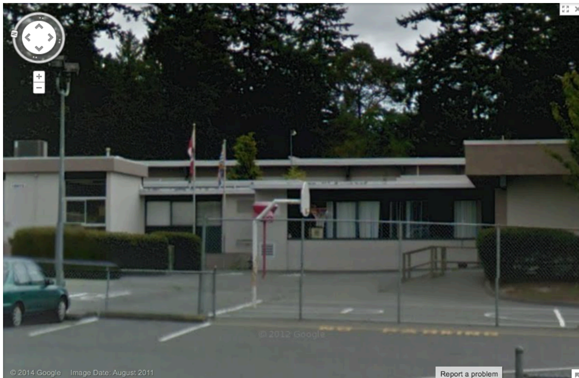
Figure 3.5: A weather station mounted on the roof of Deep Cove Elementary School (Stn. ID 62) (Google Maps 2014e).
