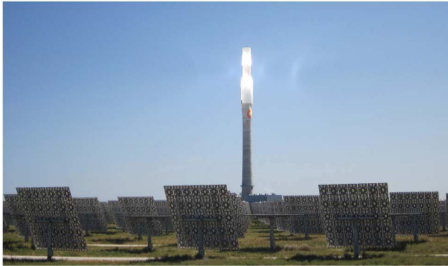
Figure 8: Gemasolar power plant in collection mode with molten salt heated at the illuminated receiver
