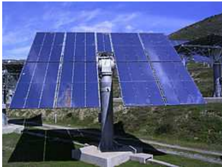
Figure 7: Mirror modules interconnected to form heliostat
