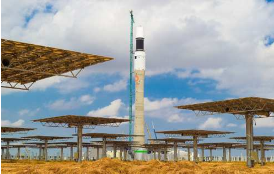
Figure 10: External receiver at Gemasolar
