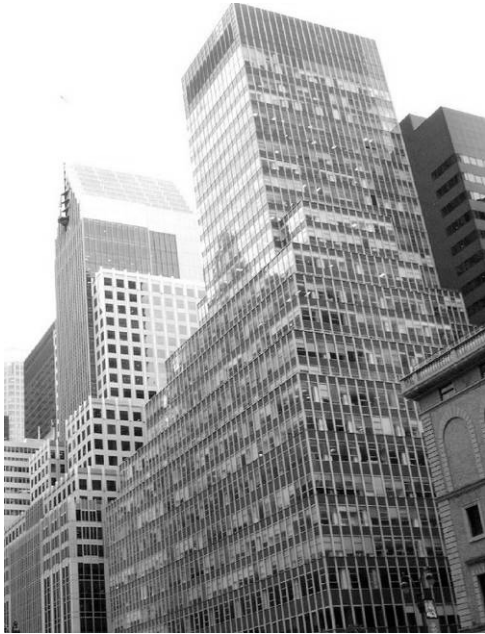
Fig.1.4. View of Park Avenue looking south, with generic glass office towers.
