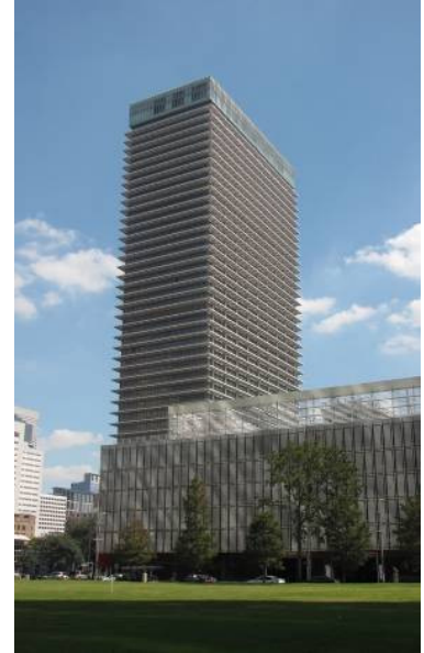
Fig.2.22. The ExxonMobil Building by Welton Becket and Associates, built in 1963. Has been sold and is going to be re-skinned.
