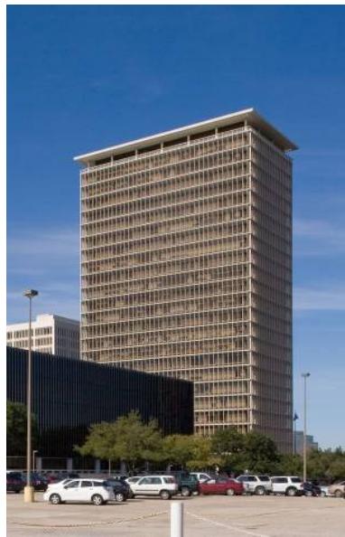
Fig.2.21. The Wortham Tower known for its deep set windows and brise-soleil. Built in 1965 by Lloyd Morgan and Jones.
