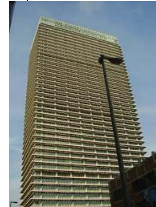
ExxonMobil Building Houston
