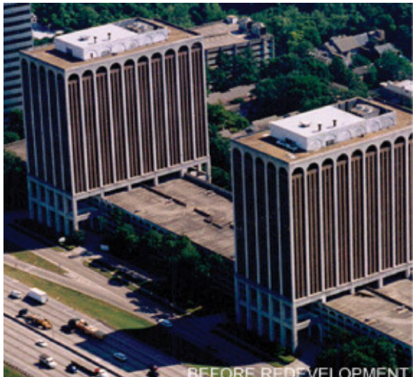
Fig.2.13. Park Towers was re-skinned after being vacant for ten years. It took on a new façade with a double glazed blue curtain wall. This was a real estate decision, as the new façade increase the floor area of the building and gave it a new appearance.
