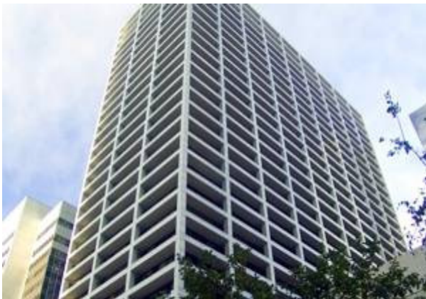
Fig.2.10. One City Centre which was originally First City Bank, had marble cladding on the external skeleton, which had deteriorated and was falling. It was re-clad with granite which is less porous therefore more durable.
