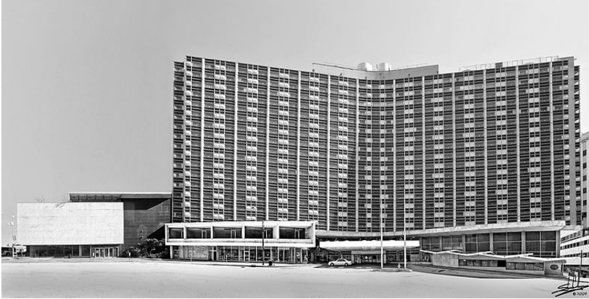
Fig.1.6. Staler Hilton in Dallas has been an endangered modern building for several years. The curtain wall has porcelain enamel panels.
