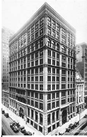
Home Insurance Building Chicago
