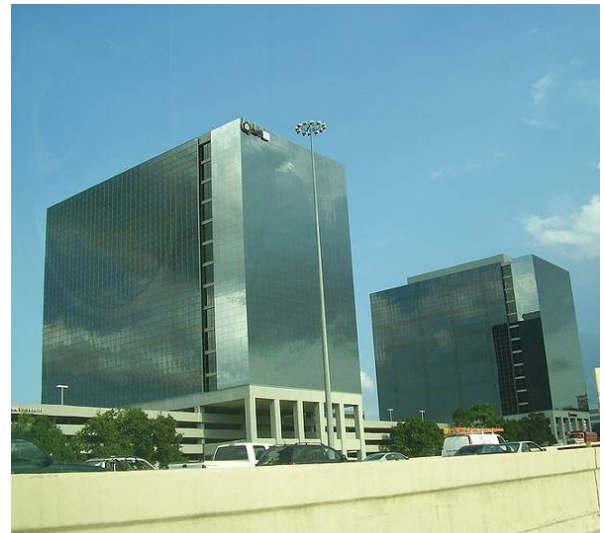
Fig.2.13. Park Towers was re-skinned after being vacant for ten years. It took on a new façade with a double glazed blue curtain wall. This was a real estate decision, as the new façade increase the floor area of the building and gave it a new appearance.
