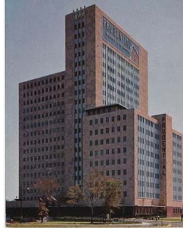
Prudential Building Houston
