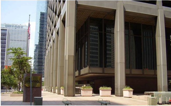
Fig.2.9. The Tenneco Building now the KinderMorgan Building underwent its first major renovation after 40 years. The Image on the left is before the renovation and the image on the left is after. The elevated lobby did not have a sufficient ground presence, and it was wrapped with a curved glass curtain wall.
