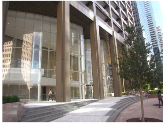
Fig.2.9. The Tenneco Building now the KinderMorgan Building underwent its first major renovation after 40 years. The Image on the left is before the renovation and the image on the left is after. The elevated lobby did not have a sufficient ground presence, and it was wrapped with a curved glass curtain wall.
