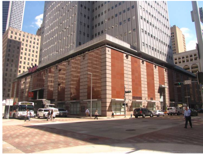
Fig.2.7. 919 Milam was initially owned by Bank One. Image on the left shows an early rendering of the building. Image on the right shows changes made to the podium. The completely red granite clad podium of 919 Milam was broken with vertical strips of grey granite that expressed the inner columns of the building. Here the red granite was removed and reused in place. The more post-modern modification of the faced is not considered authentic to the starker original modern façade.
