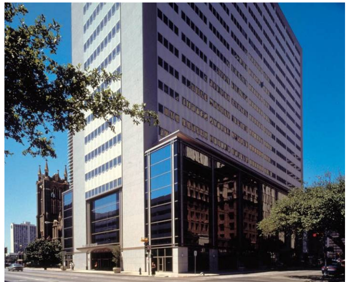
Fig.2.8. The first five floors of the Travis Tower were re-skinned. The challenge here was to conduct the façade change while the tenant still occupied the spaces.
